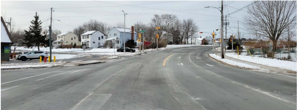
Woodlawn Road at Settle Street and Valleyfield Road looking west
