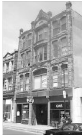
Victorian Gothic/Art Nouveau G.M Smith Building
