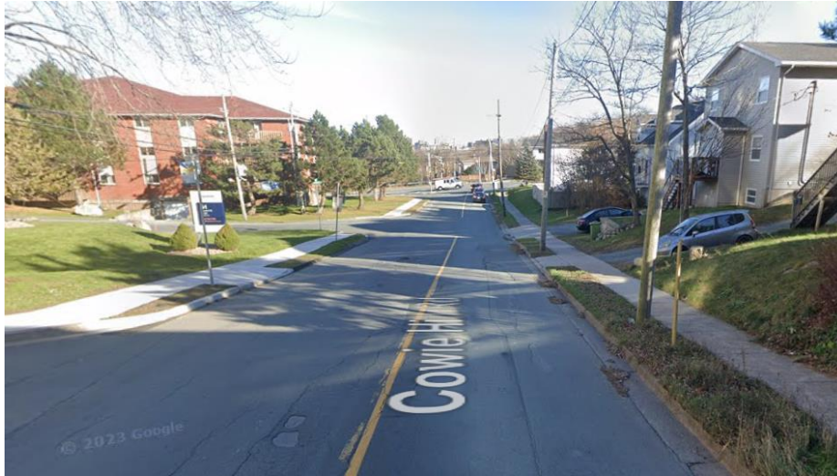
Figure 4 - Cowie Hill Road towards Herring Cove Road
