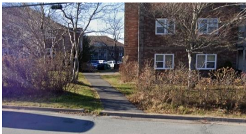
Photo 1: Pedestrian Walkway Discontinuity at 68 Mountain Road
