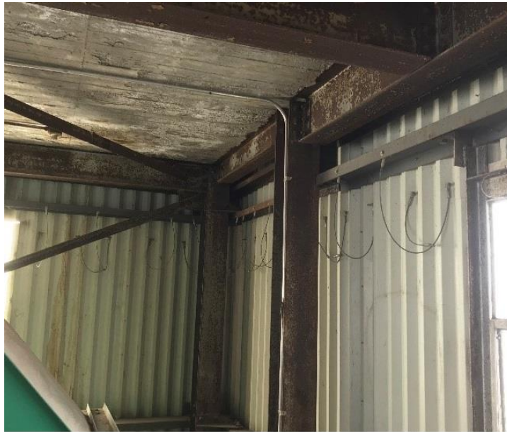
Figure 3.2: Photograph of the explosion release cladding on the exterior walls in Workhouse #3.
