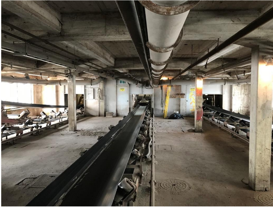
D.17: Partition between Annex 1 and Annex 2.
