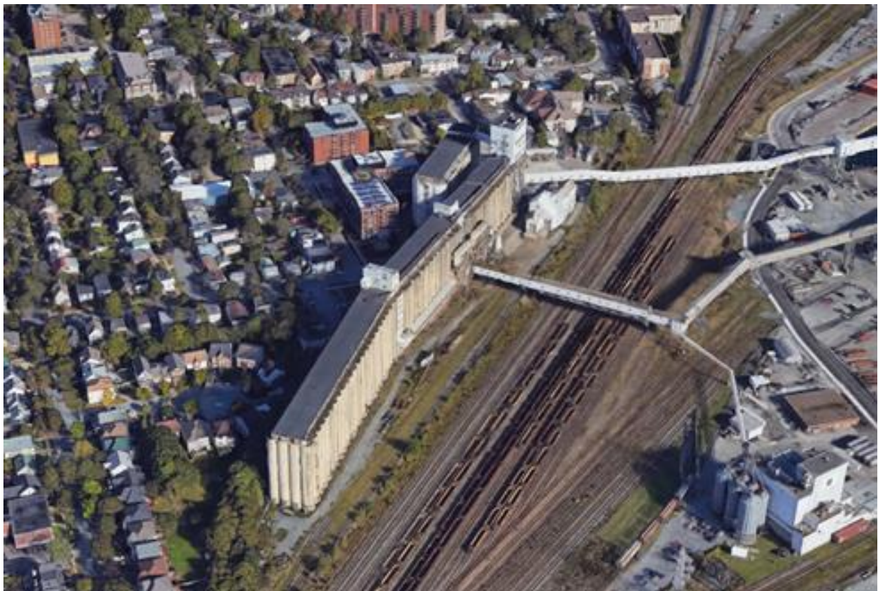
Figure 2.1: Image of the grain elevator site facing north (obtained from Google Earth).
