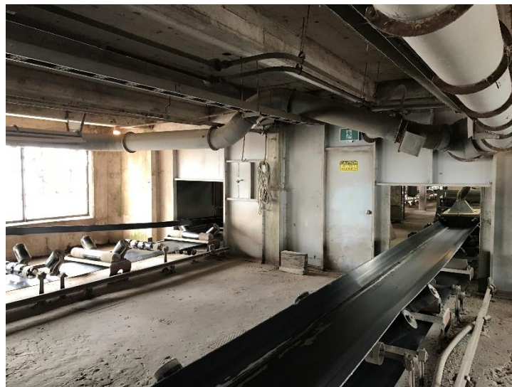
Figure 3.3: Photograph of partition located between Annexes 1 and 2.
