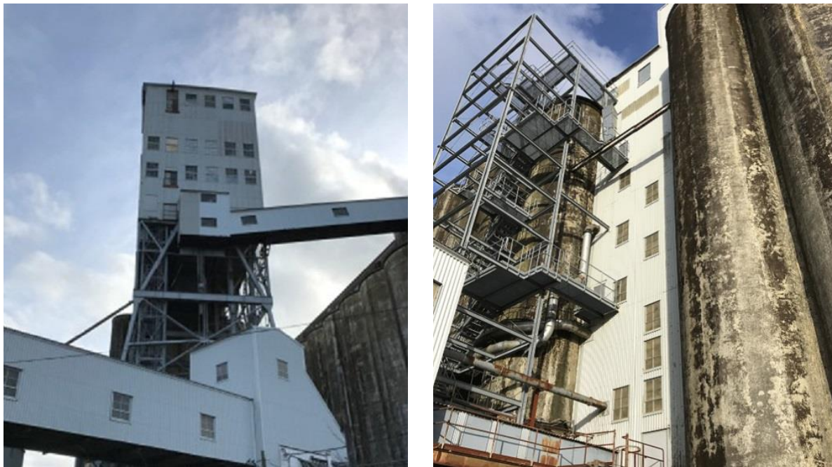
Figure 2.7: Workhouse #1 tower (left) and Workhouse #2 area (right).
