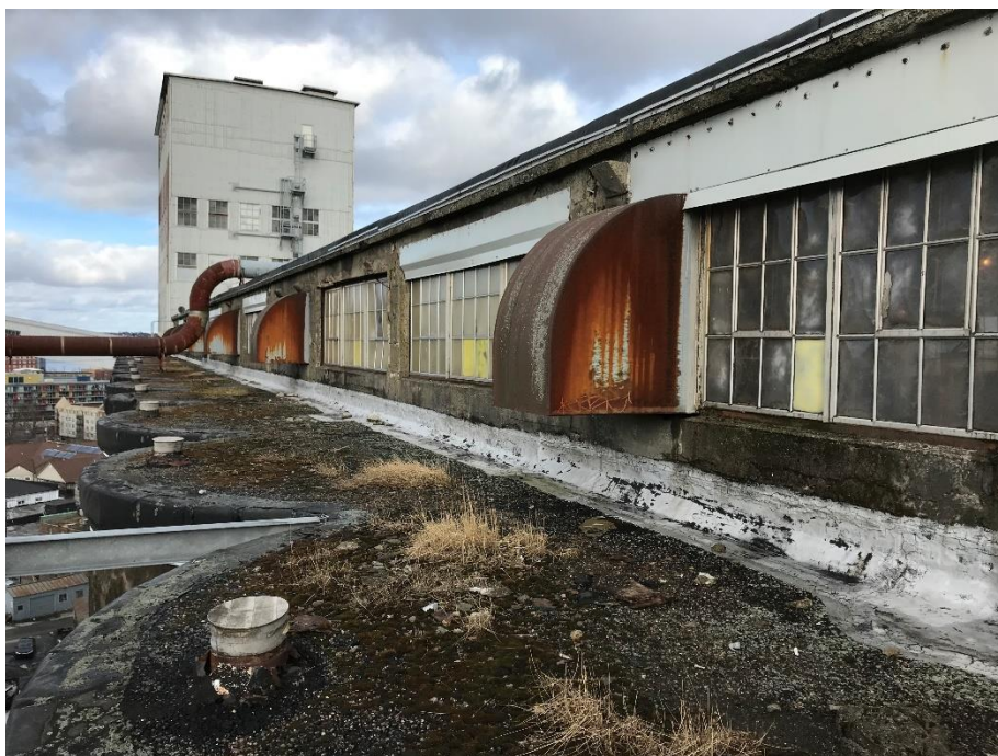
D.4: Exterior of Annex 1 bin level gallery (western side).
