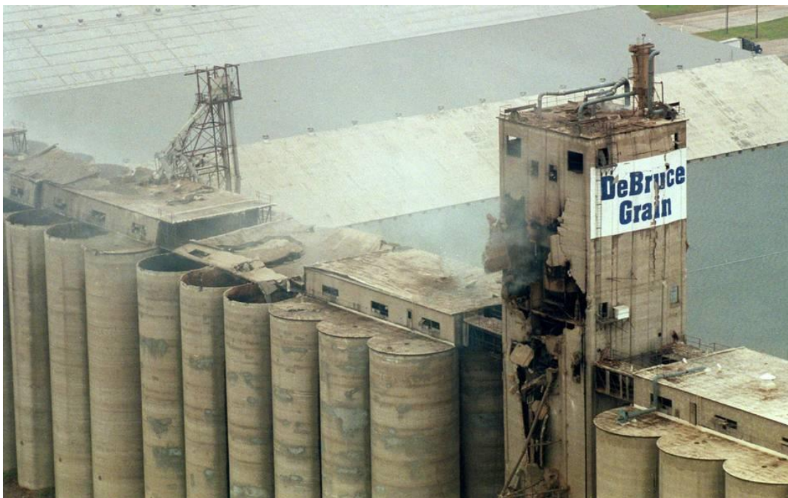
Figure 6.6: Resulting damage to the DeBruce grain elevator.
