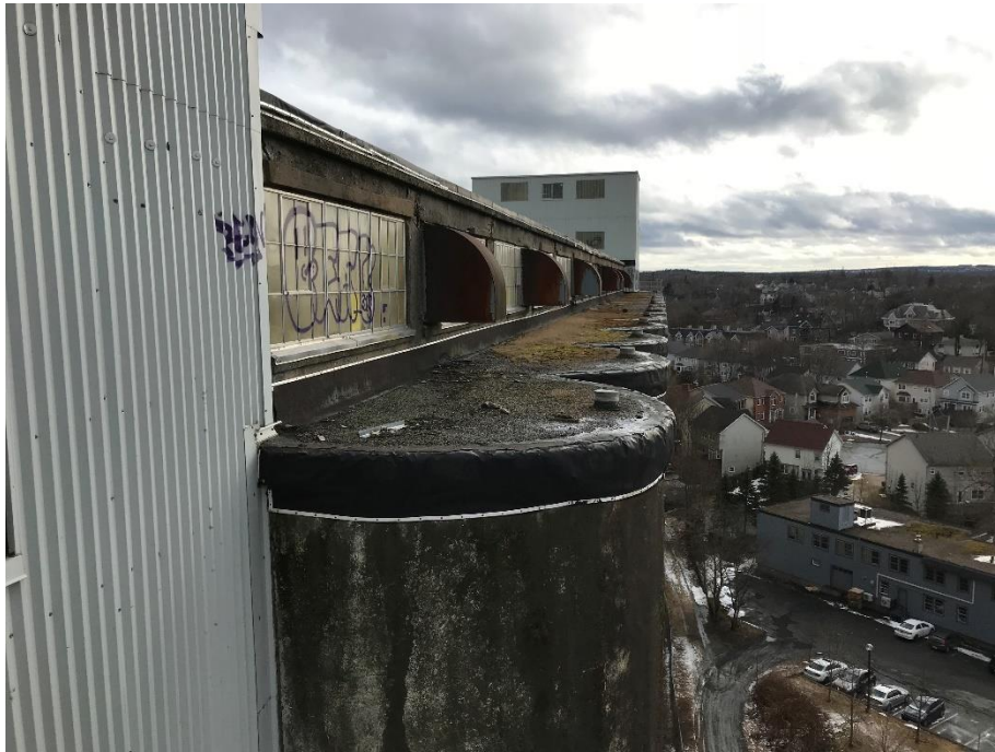
D.5: Exterior of the Annex 2 bin level gallery (western side).
