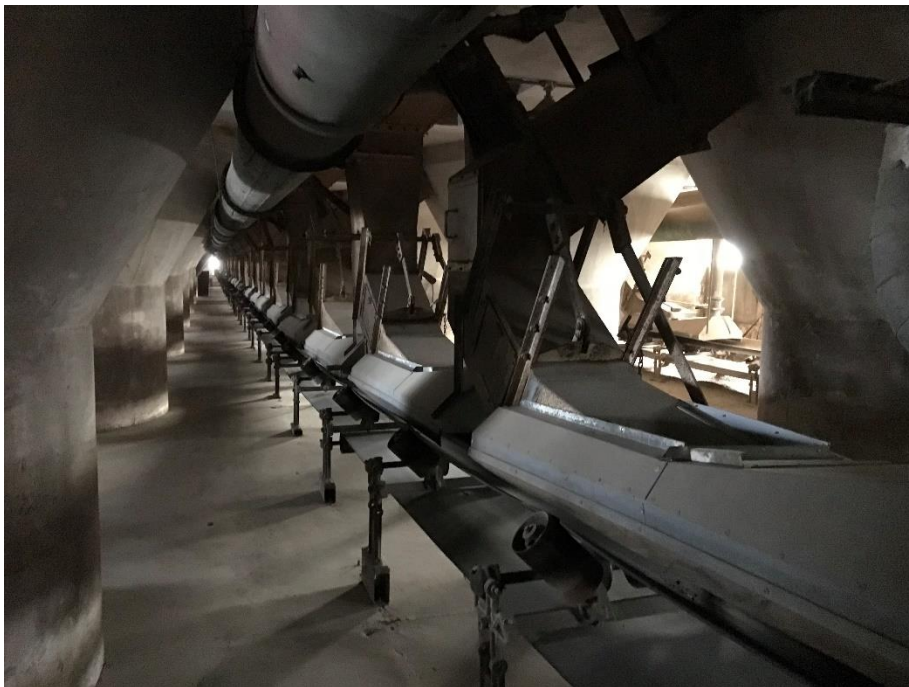
D.20: Annex 3 basement level gallery.
