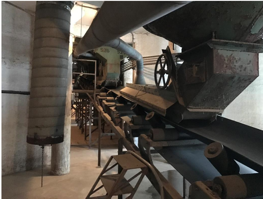
D.11: Annex 4 basement gallery.
