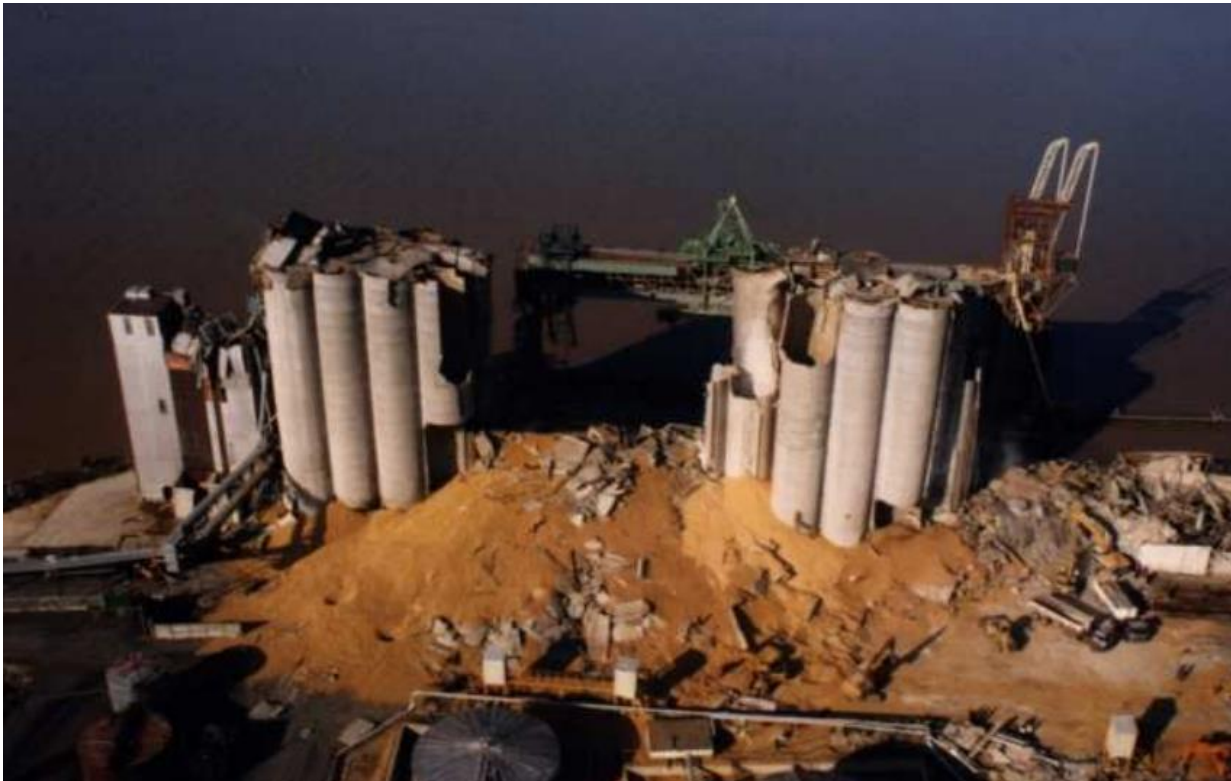
Figure 6.4: Resulting damage to the SEMABLA grain handling facility following the dust explosion event.
