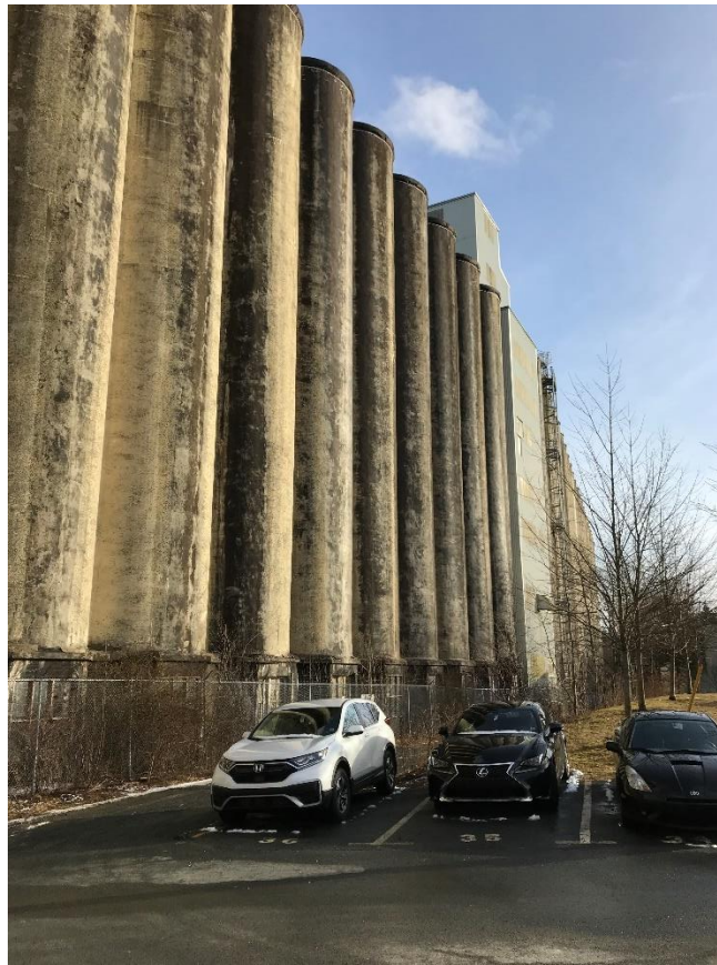
D.8: Western side of Annex 2 silos and Workhouse #3.
