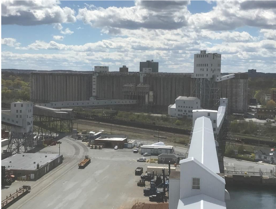
D.1: Photograph of the facility from the marine tower (east side).
