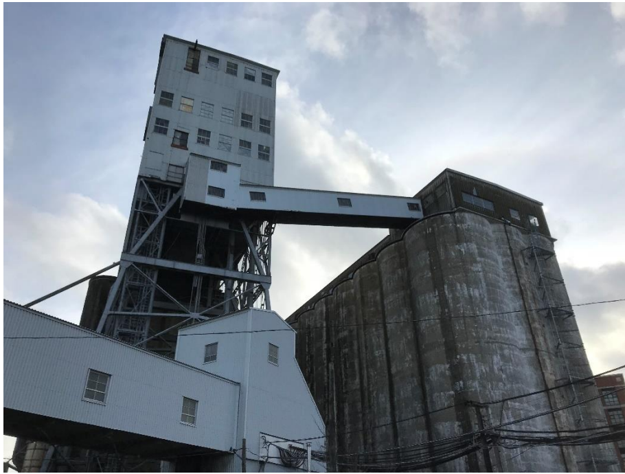
D.7: Workhouse #1 and Annex 4 (looking south).
