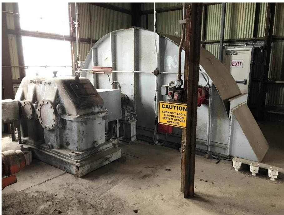
D.22: Bucket elevator head in Workhouse 1 motor floor.
