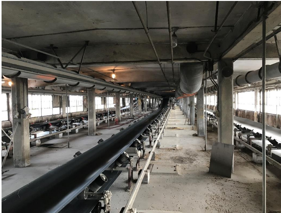
D.15: Annex 2 bin level gallery.
