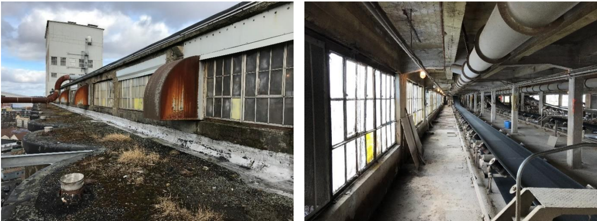
Figure 2.5: Exterior (left) and interior (right) of the Annex 1 bin level gallery.
