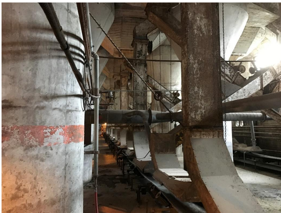
D.16: Annex 2 basement gallery.
