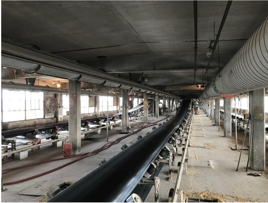
D.19: Annex 3 bin level gallery.
