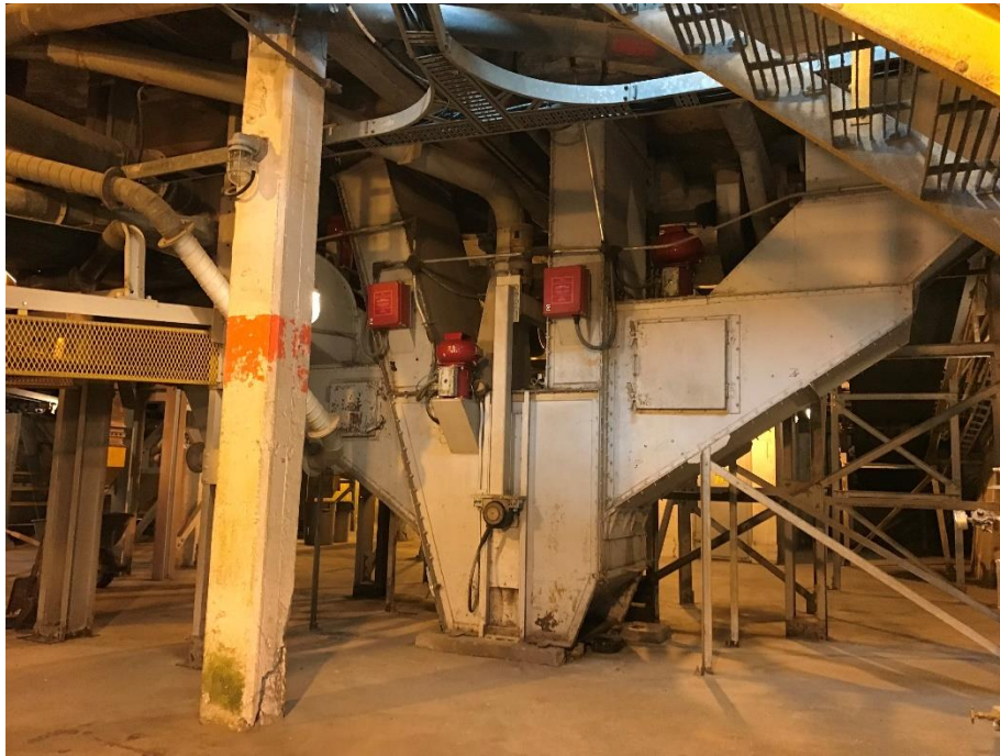
D.21: Bucket elevator boot in Workhouse 1 basement.
