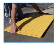
Fast, easy installation with included adhesive and anchor system. Apply adhesive to scored areas on back, place in desired location and install anchors
