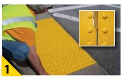
After ensuring "General Conditions" (refer to box on left) have been met, and surface has been properly cleaned, place mat(s) in desired final position. If mats are placed side by side, leave a 1/8 in. gap between them.
