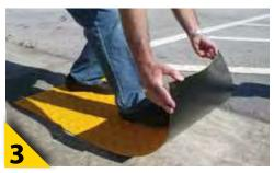
Roll and press the exposed portion onto the surface. While standing on the attached end, peel the remaining sections of the backing and press and roll onto the surface.
