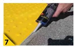
Cut the nozzle of the sealant tube at the 1/4 in. mark. Apply a smooth, thin bead of sealer around the perimeter (sealer is not required between adjoining mats). Mats are ready for immediate use once installation is completed and edge sealant has dried to the touch. Tip: To make the edge sealer dry faster, mist with plain water.
