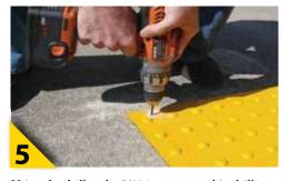
Using the drill and a 5/32 in. masonry bit, drill through the pre-drilled holes into the concrete to a depth of 1 1/4 in. If the mats are trimmed so a predrilled hole is removed, a new hole must be drilled in the mat using a 3/8 in. standard drill bit, 2 in. from the side edge and 1 in. from the beveled edge.
