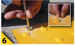
Be sure the screw and the matching washers are oriented so the neck of the screw falls into the inside taper of the washer. Using a phillips screwdriver, fasten the screws into the drilled holes. The proper screw tightness will allow a slight finger twist of the washer. Do not overtighten.
