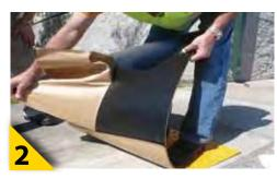
While standing on the mat to prevent movement, remove one section of the paper backing.
