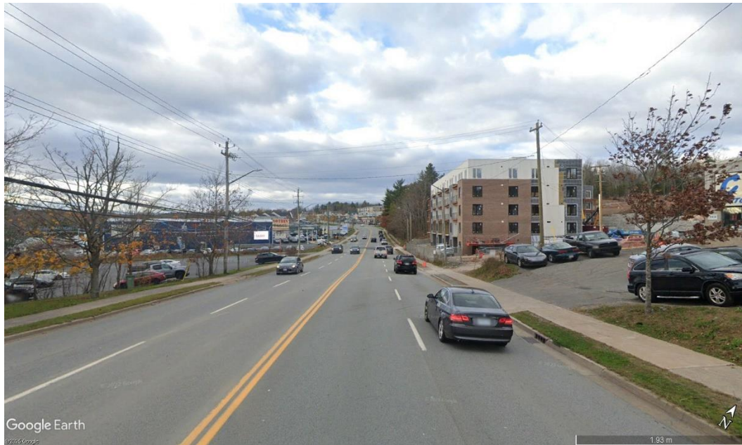
Figure 3 - Sackville Drive Looking North
