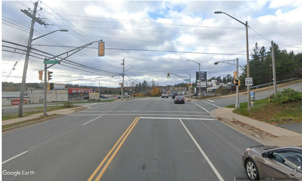
Figure 5 - Sackville Drive at Armoyan Drive.
