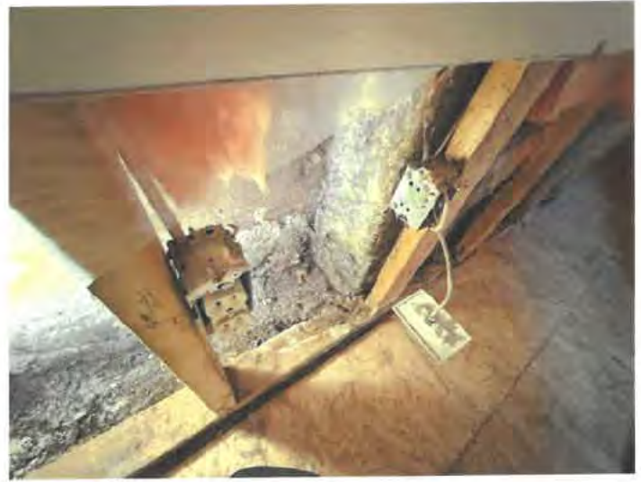
Photo No. 6 – Efflorescence and wood rot at interior wall to foundation location.
