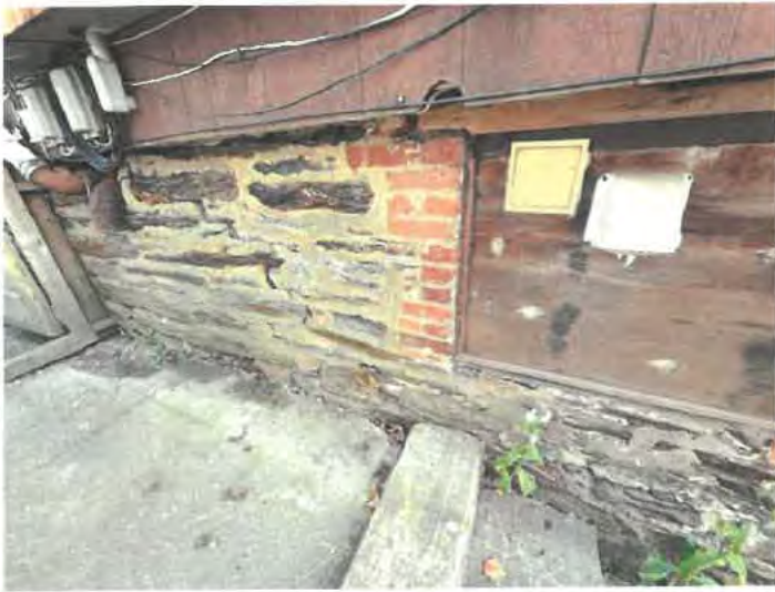
Photo No. 1 – Stepped settlement and wall deterioration in stone masonry.
