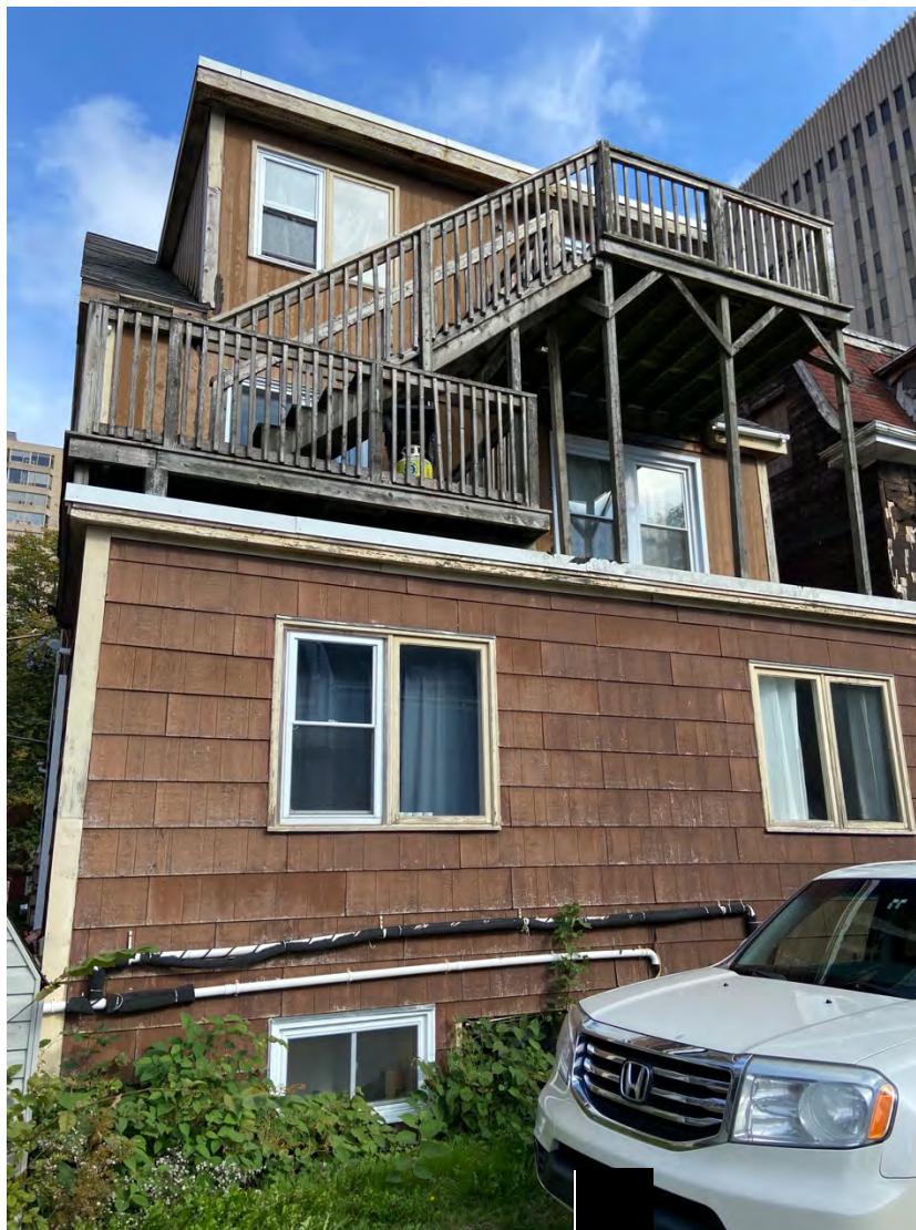
Figure 48: Extension to the main floor and basement, and attic shed dormer with fire escape at the rear of 1460 Carlton Street
