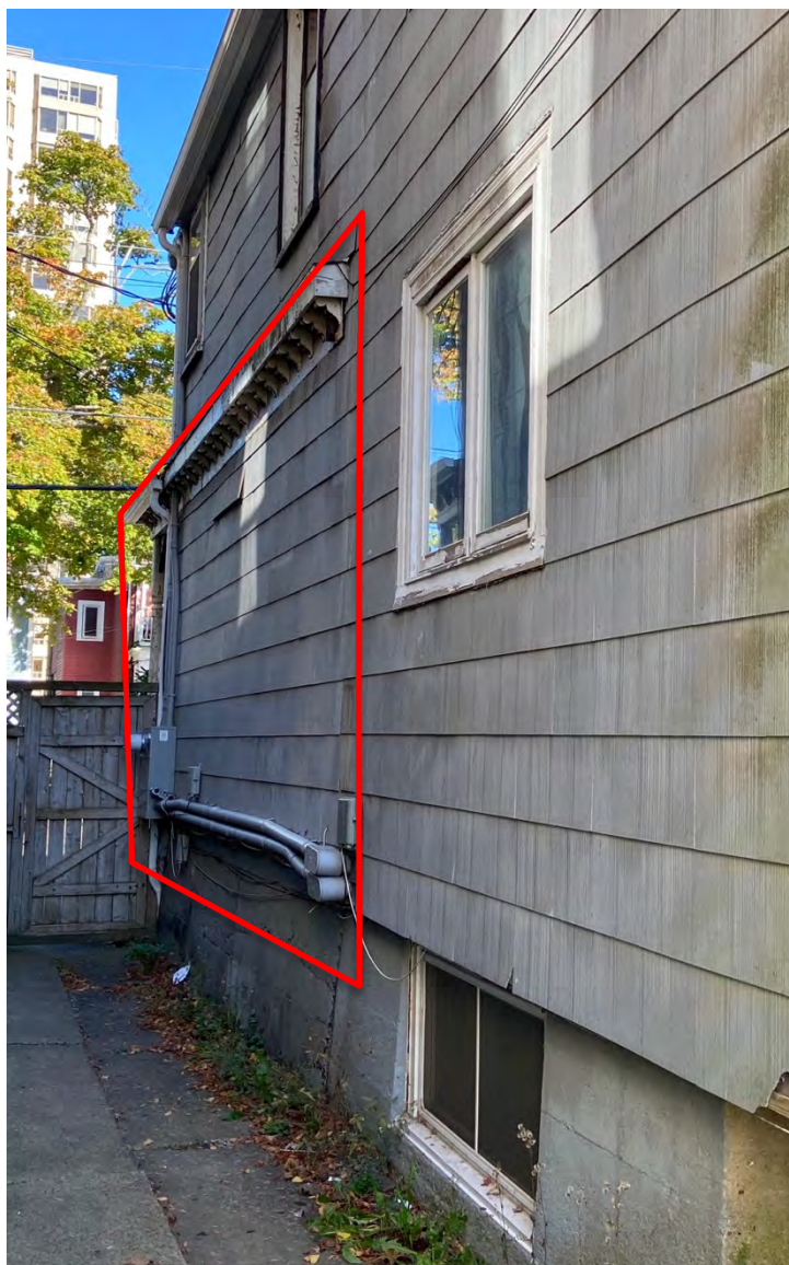
Figure 56: Remnants of wrap-around porch (roof line and brackets), and full extent of that side of porch outlined, north side
