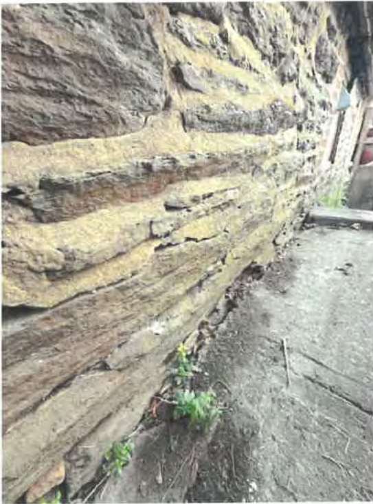
Photo No. 5 – Deteriorated stone masonry with open mortar joints and inward lean into basement.
