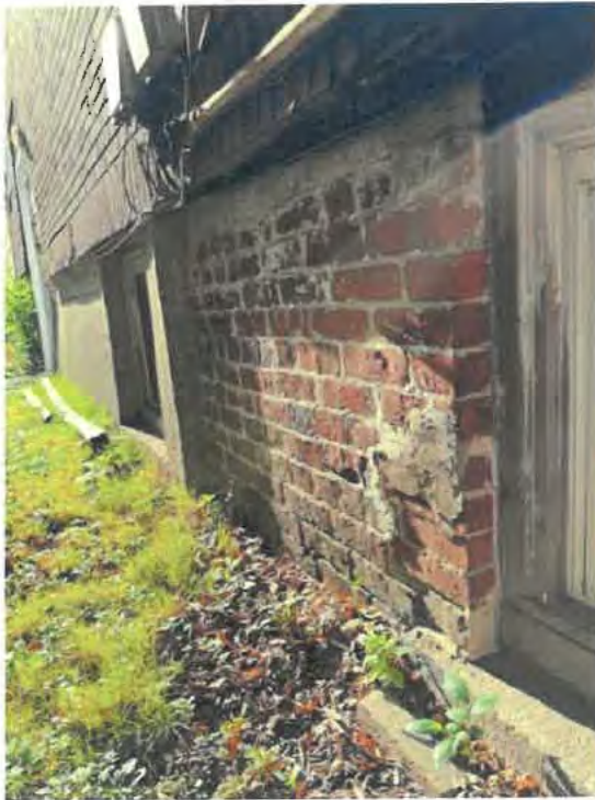
Photo No. 3 – Deteriorated brick masonry. Inward movement at grade. Concrete added to wall face in background.
