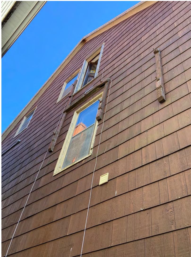
Figure 46: Shingle pattern on north side and alterations to accommodate former fire escape including a door in the attic
