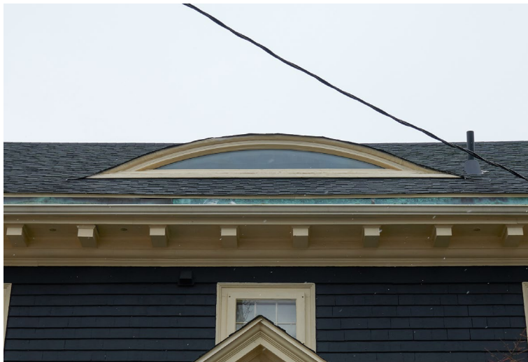
Figure 19: Cornice with dentils, copper eavestrough, and the eyebrow dormer window (March 2025)
