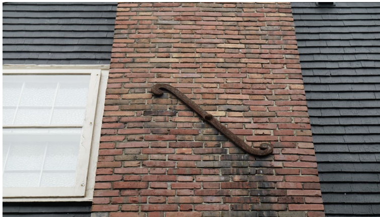
Figure 18: Anchor plate on the brick chimney (March 2025)
