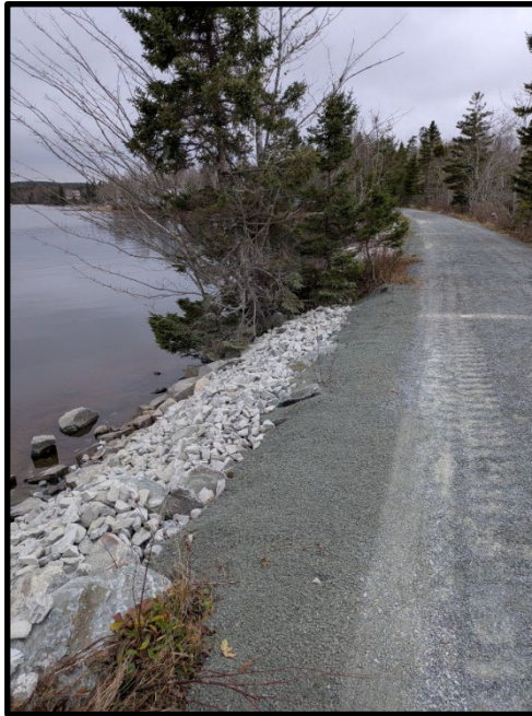
Gaetz Brook Greenway SATA Trails Society Embankment Stabilization
