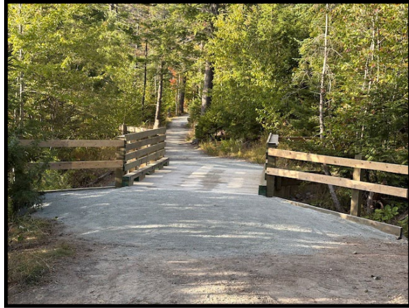
First Lake Glen Sleunwhite Trail Friends of First Lake Society Bridge Replacement
