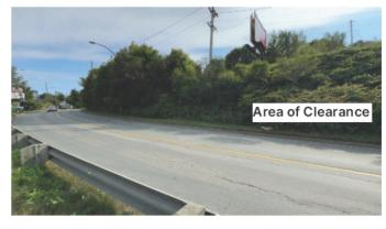
Sight distance implications to the south are shown in the image to the right. Field measurements show an existing sight distance to the east of about 75 meters and is restricted by existing roadside vegetation.
