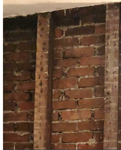
Ballon-like construction evident in spacing of studs with nail marks
