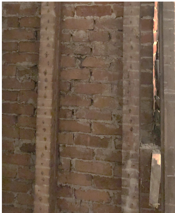
Figure 13: Image of striped interior wall in Porters House, showing lighter uniform studs with nail marks showing utilization of lighter balloon style framing methods (Image from applicant)
