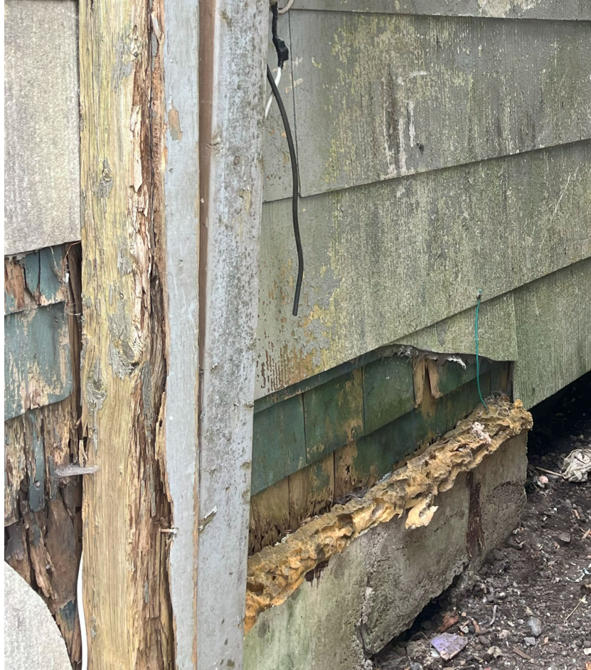
Figure 20: Photograph of siding on north elevation of 2320 Maynard showing underneath new vinyl siding (Staff visit, September 19 th , 2024)
