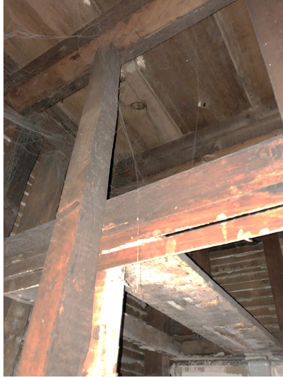
Figure 12: Image of interior foundation of Porters House during interior work, showing timber framing style (Provided by applicant)
