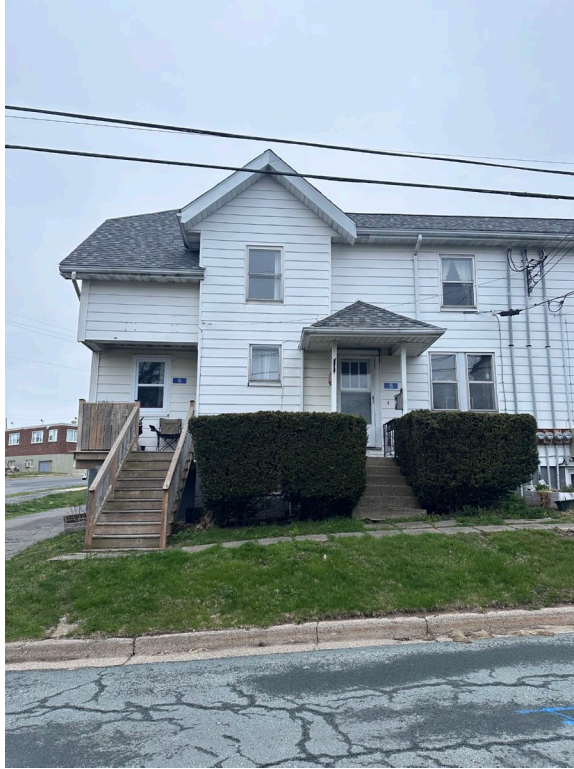
Figure 26: Entrances to 6 and 8 Ropewalk Lane (May 1, 2024)
