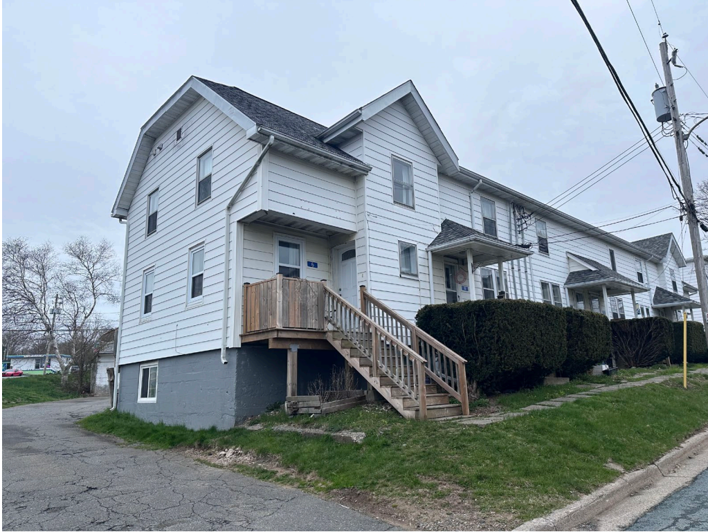
Figure 22: South and West Elevation of 6 to 16 Ropewalk Lane (May 1, 2024)
