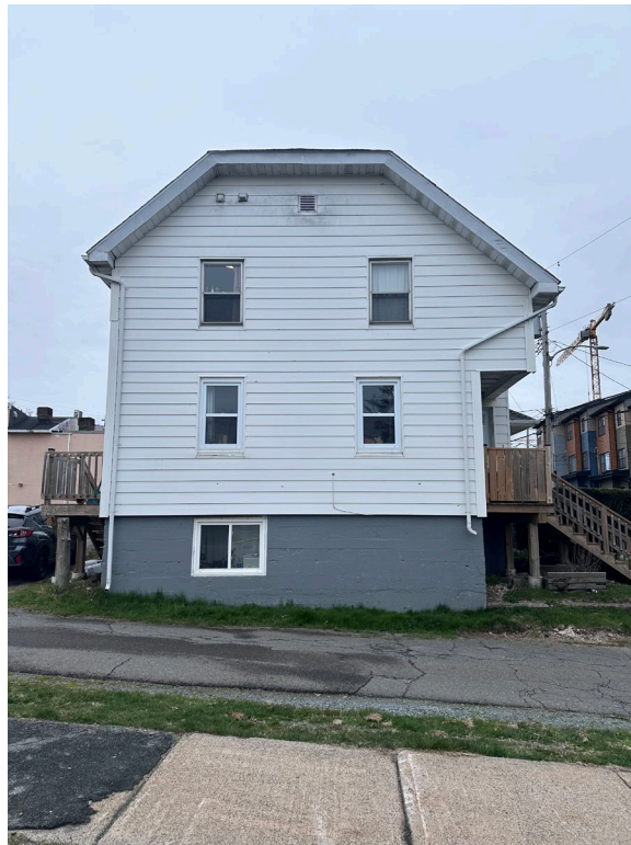
Figure 23: West elevation of 6 to 16 Ropewalk Lane (May 1, 2024)
