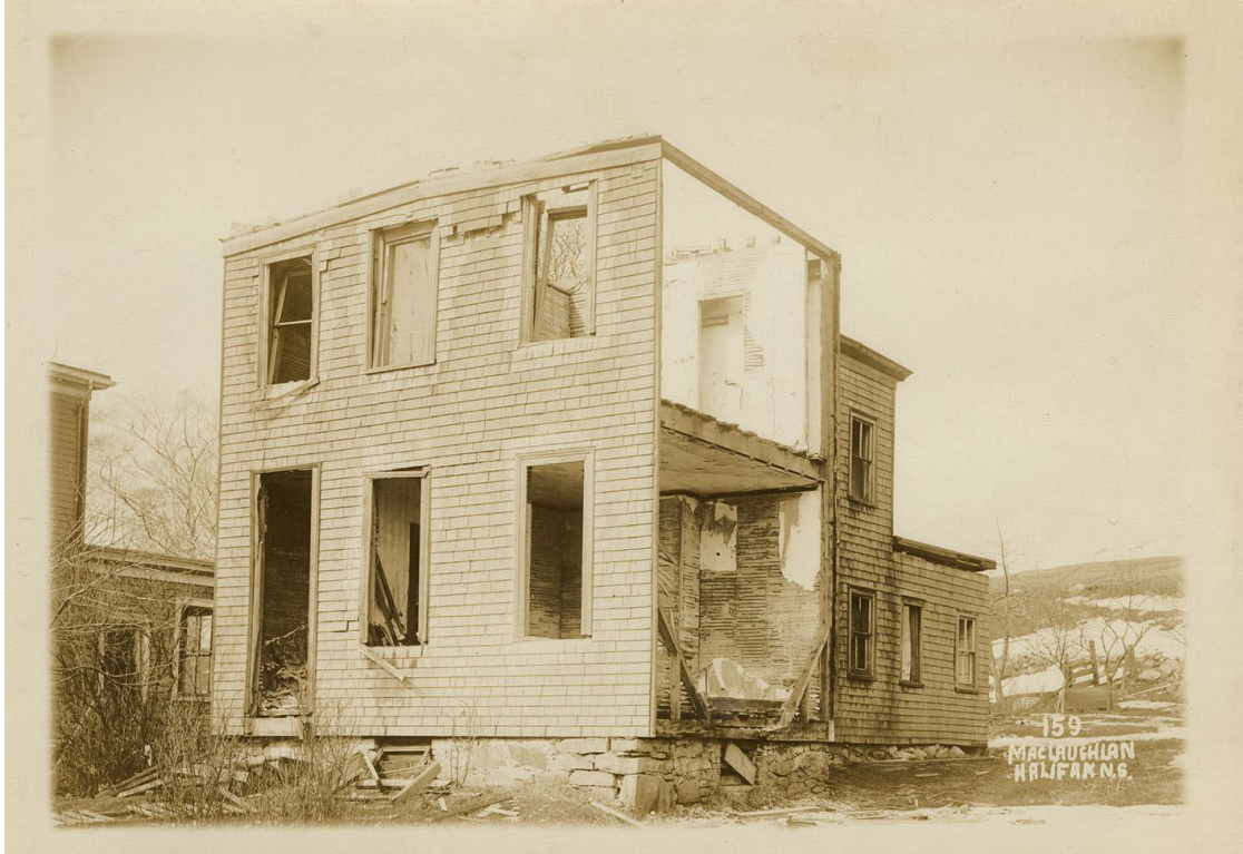
Figure 30: A damaged house on Hester Street, of similar style to 20 Ropewalk Lane (MacLaughlan, Album 2, No 159).
