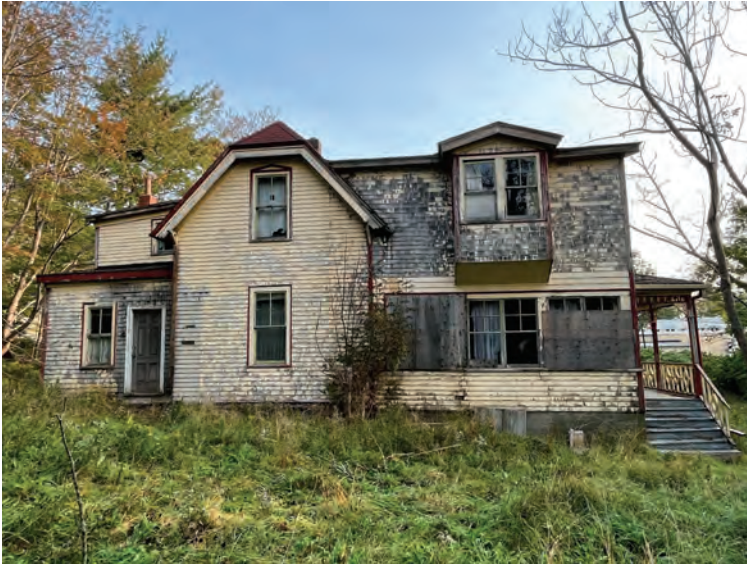
South side with remainder of porch
