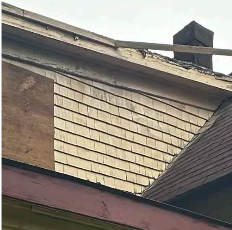
Figure 13: Chimney located on the rear of the house, facing west elevation (Staff photo, July 17th, 2024)
