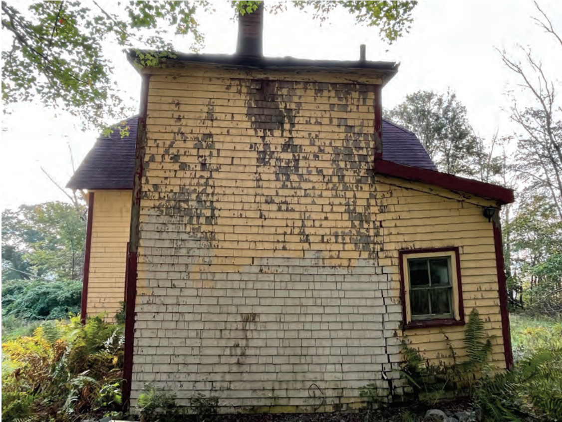
Figure 18: Rear of house
