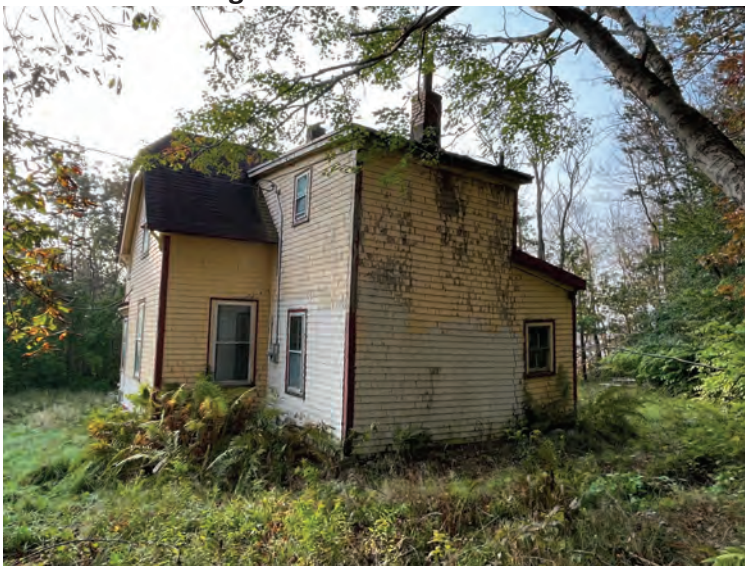
Rear addition protruding out from the 1917 addition.
