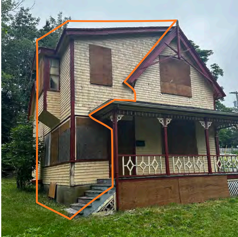
Figure 21: Red Gables from south elevation with circa 1934 upstairs and enclosed porch addition outlined in orange (Staff photo, July 17 th , 2024)
