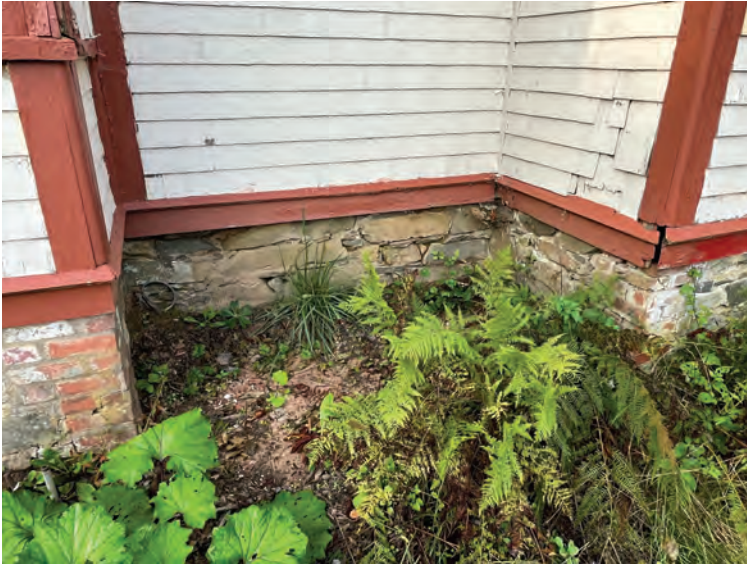
Stone and brick foundation on north side
