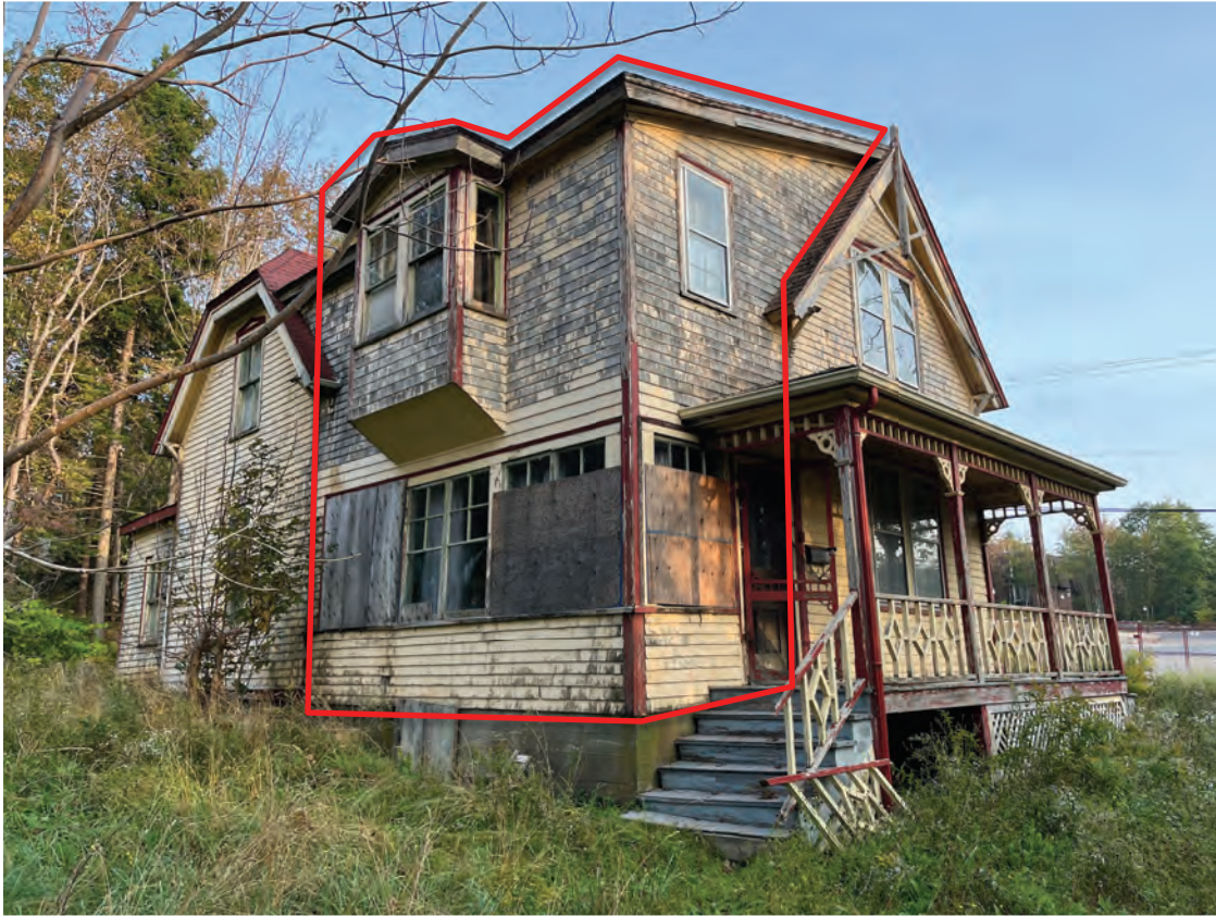
Figure 26: Shed roof extension on south side outlined.
