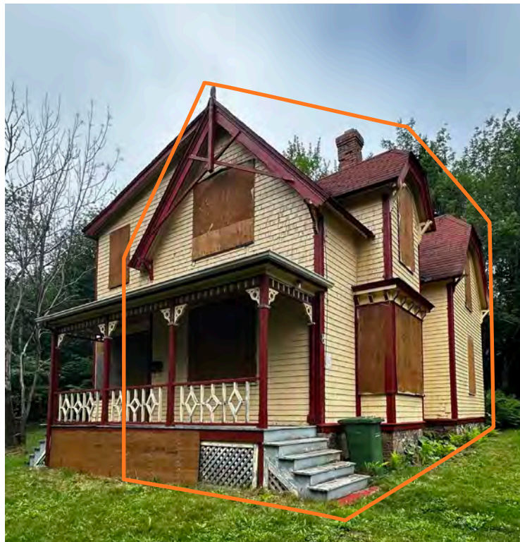
Figure 22: Red Gables North elevation with likely original structure outlined in orange (Staff photo, July 17 th , 2024)
