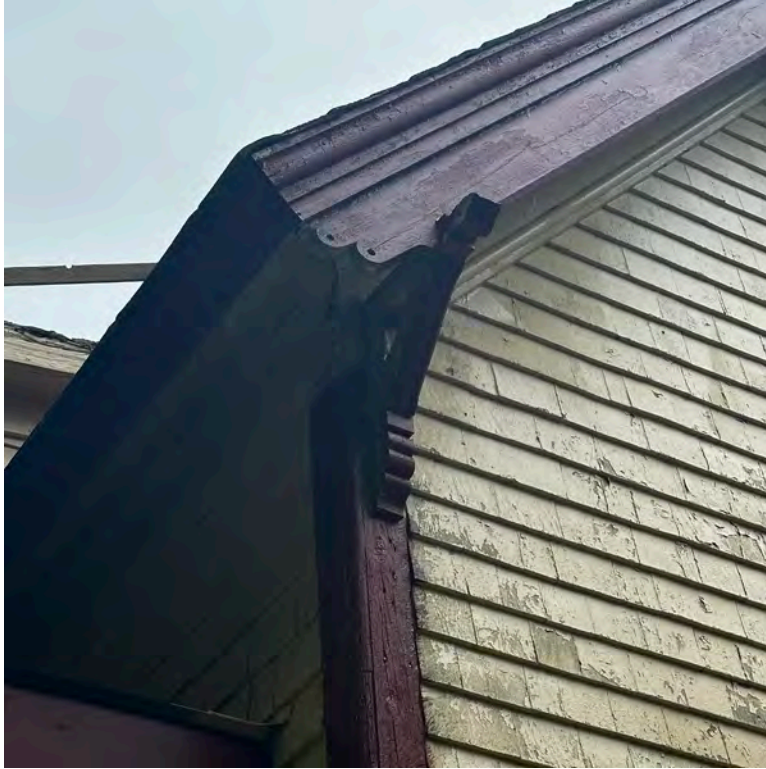
Figure 14: Brackets and molding on front gable verges (Staff photo, July 17th, 2024).
