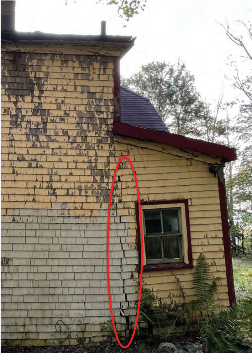
Figure 25: Separation occurring in the rear wall face as a result of settling.
