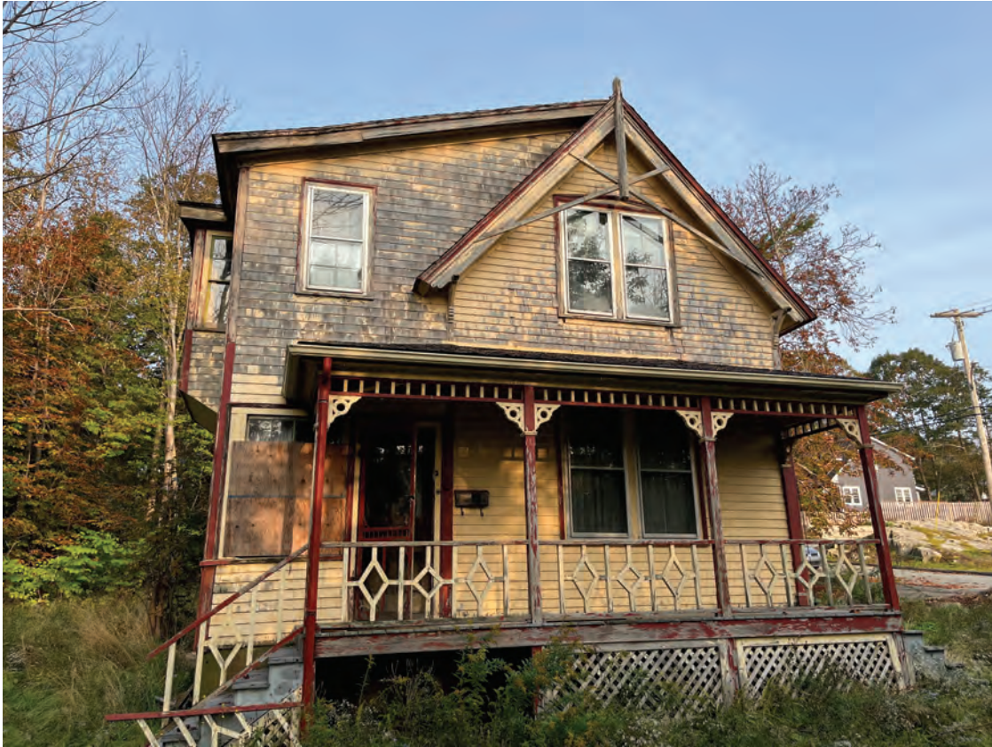
Figure 15: Front of house, east side
