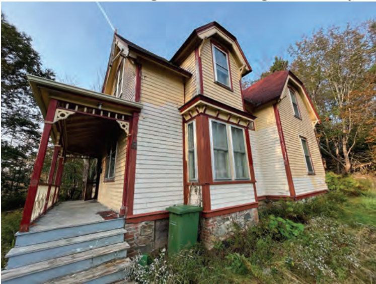
North side showing the front porch as part of the c. 1870 house and its 1917 addition to the right.
