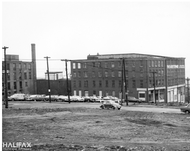
Figure 18: Portion of Clayton & Sons factory building on Jacob Street ca. 1966, demolished for urban renewal (Source: Halifax Municipal Archives)
