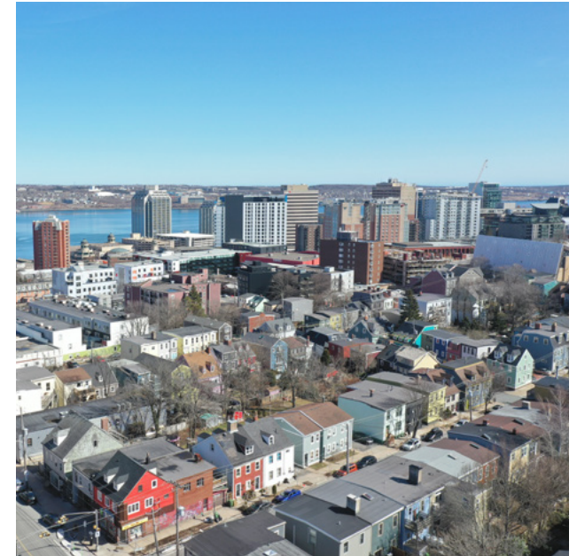
AERIAL VIEW LOOKING TOWARDS MAYNARD, CREIGHTON AND FALKLAND STREETS
