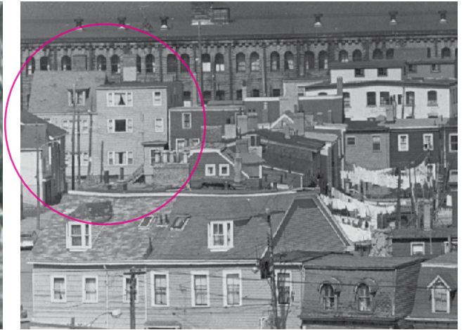
1964 - view of the Townhouses and Factory from the Citadel (detail) Note the presence of large picture windows and the staged renovation to add the third storey at 119 Cornwallis. Source: Halifax Municipal Archives)
