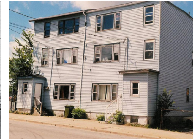
~2001 - the Townhouses from the street before the Forbes renovation. The third storey was added to the left building sometime in the 19 years between 1983 and 2002. Source: Facebook - Forbes Restoration
