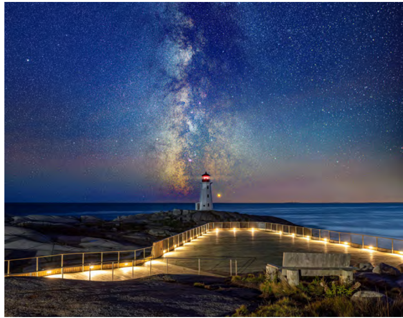
Figure 18: Under the management of Build Nova Scotia, the Peggy's Cove Viewing Platform was designed with downward directed ground level lighting to improve access and reduce sky glow (Omar Ghandi Architects, 2023).
