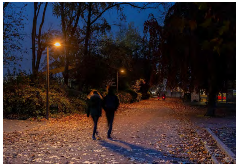
Figure 6: The City of Lille, France, is implementing ecological LED lighting parks with amber colour temperature (i.e., 2,200K - 2,700K). Motion detection sensors increase illuminance levels with the arrival of pedestrians, cyclists and cars, and return to ecological mode when there is no traffic (Schröder, 2023).
