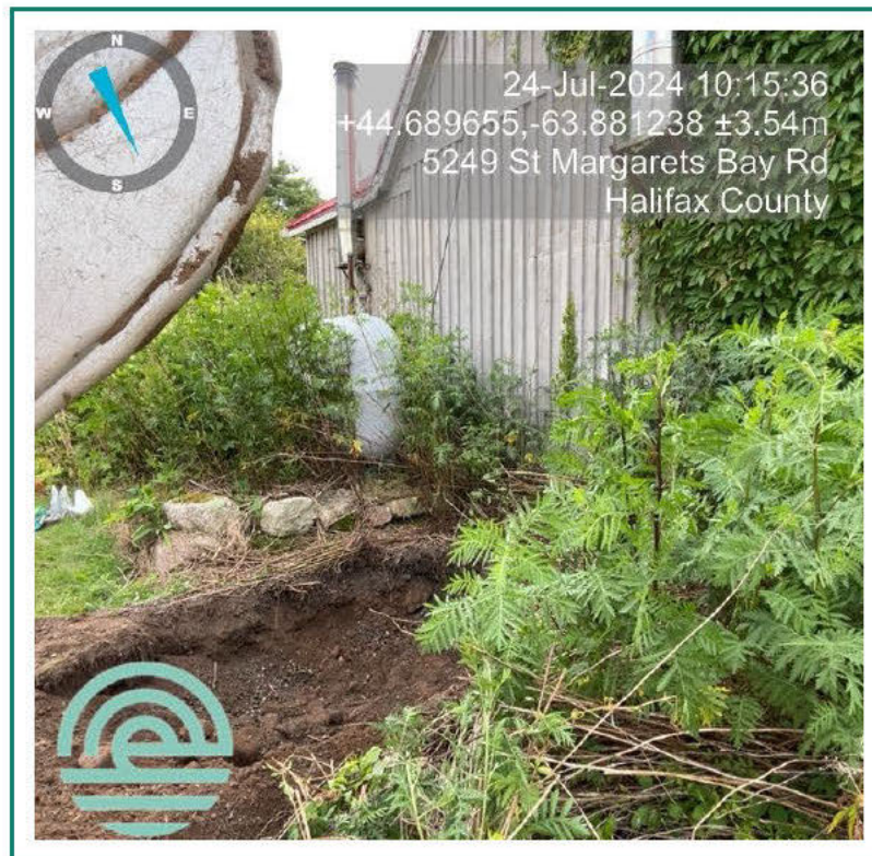
Photo 4: Photo looking northeast showing fibreglass fuel oil AST and TP1 location.
