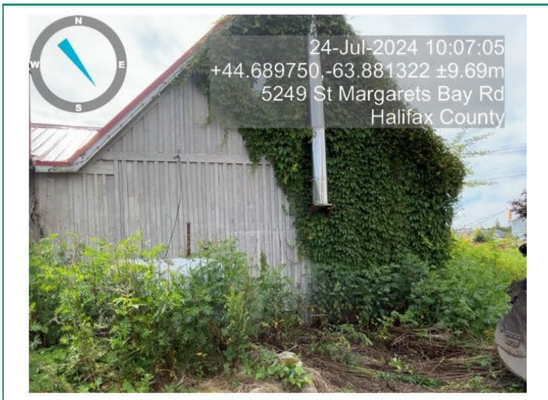
Photo 2: Photo looking southeast showing fibreglass fuel oil AST and location of old, abandoned steel AST on the west side of 5249 St. Margarets Bay Road.
