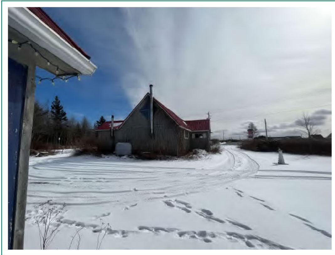
Photo 2: View (facing east) of the side of the subject building at 5249 St. Margarets Bay Rd (Feb. 28, 2023). Note the snow covered surface, exterior finishes and neighbouring buildings in the background.
