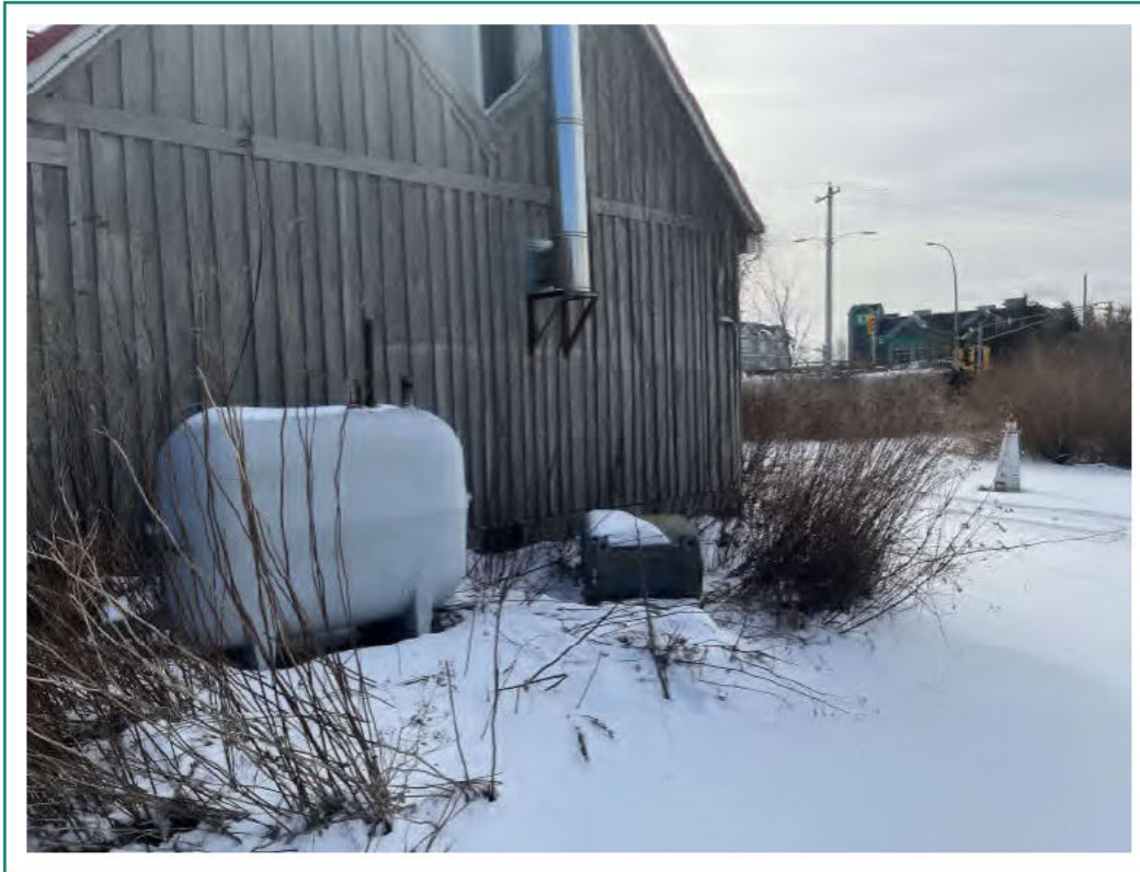
Photo 7: Photo looking south showing fibreglass fuel oil AST and the abandoned steel AST on the west side of 5249 St. Margarets Bay Road (February 28, 2023).
