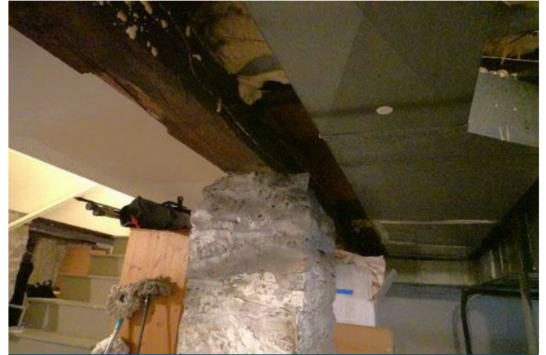
Rock foundation and wood beams in the basement
