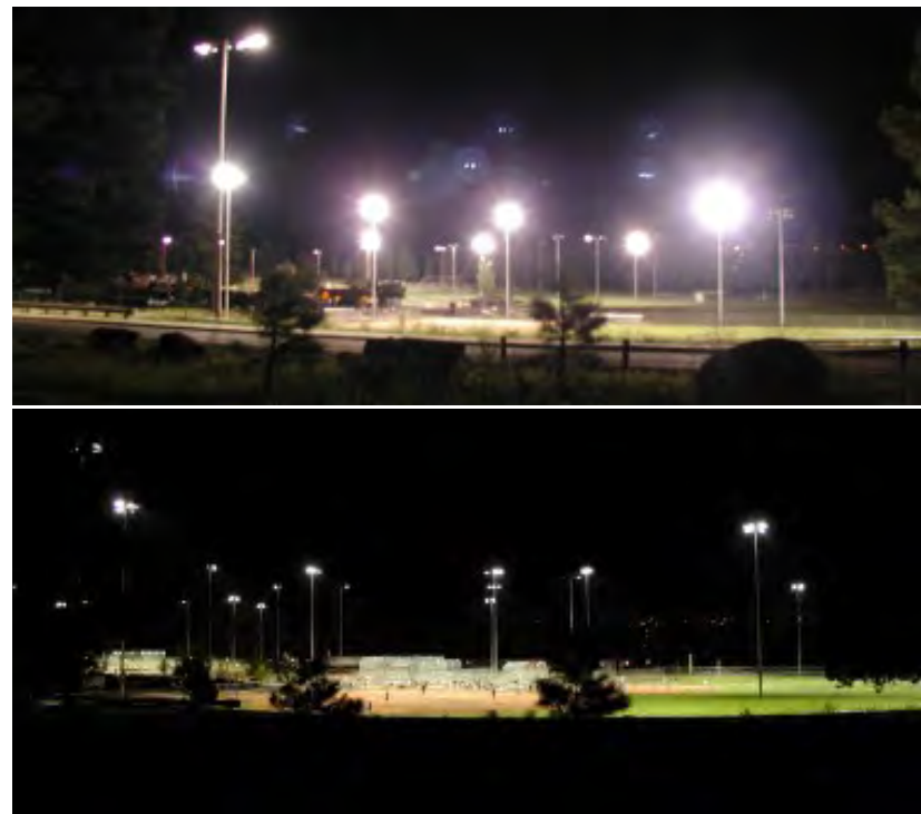
Figure 29: Lighting for sport uses can be intrusive within communities. This image illustrates the difference between shielded and unshielded sport lighting (Flagstaff Dark Skies Coalition, 2014).
