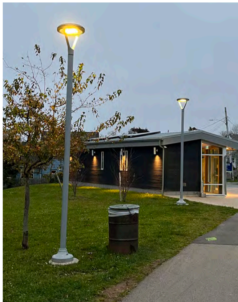
Figure 11: Park pathway lighting in Fort Needham Memorial Park is downward directed, evenly spaced, and connects destinations without gaps in lighting coverage (Cushing, 2023).
