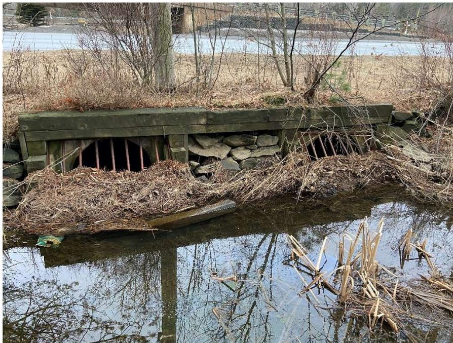
Figure 4-7: Culverts Downstream of Memory Lane
