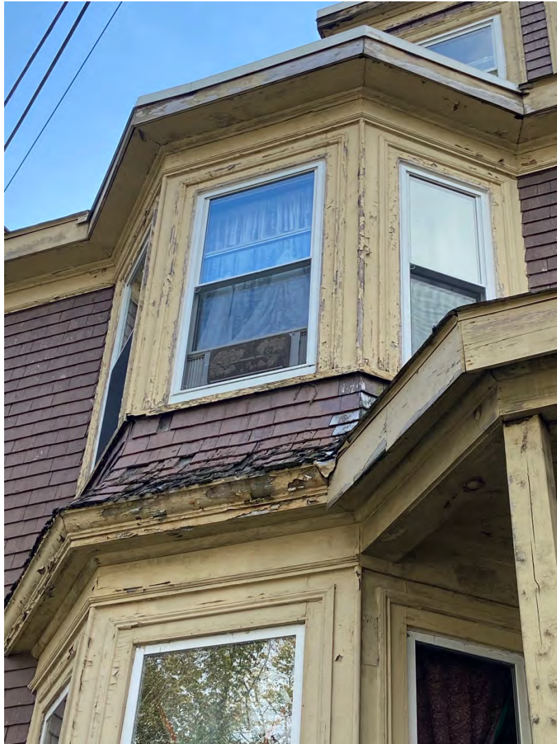
Figure 70h: Neal Residence, 1460 Carlton Street – bellcast eave
