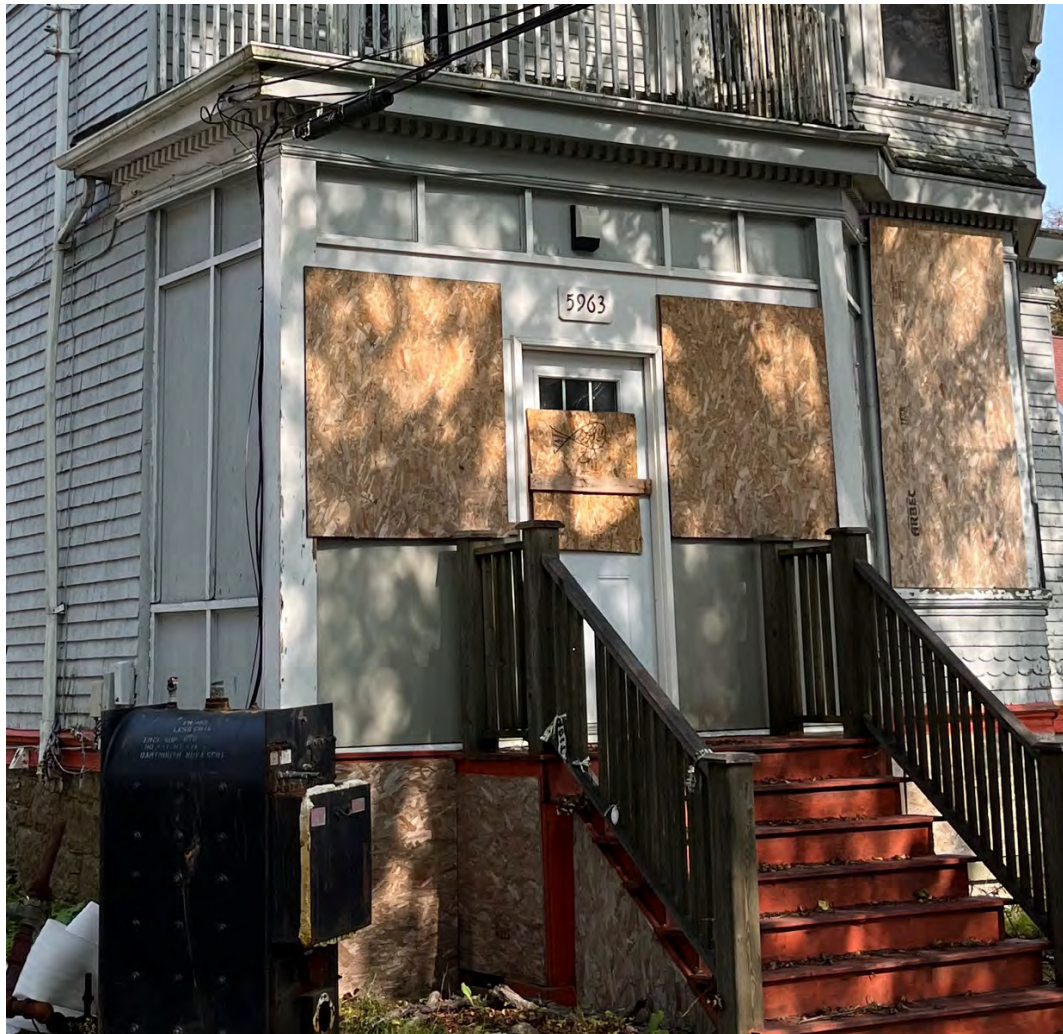
Figure 24a: Front porch enclosure of 5963 College Street
