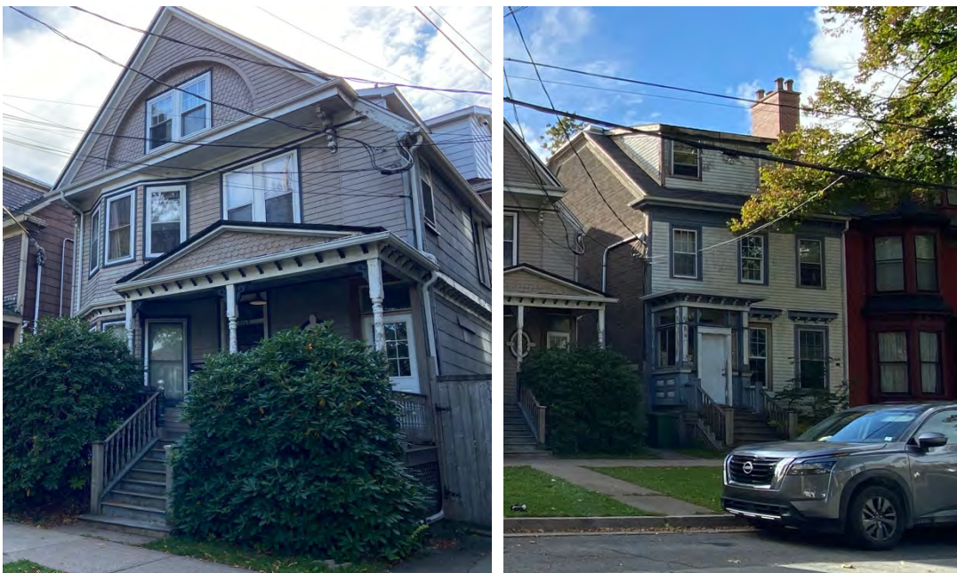
Figures 7c and 7d: 1466 Carlton Street (left) and 1468 Carlton Street (right)
