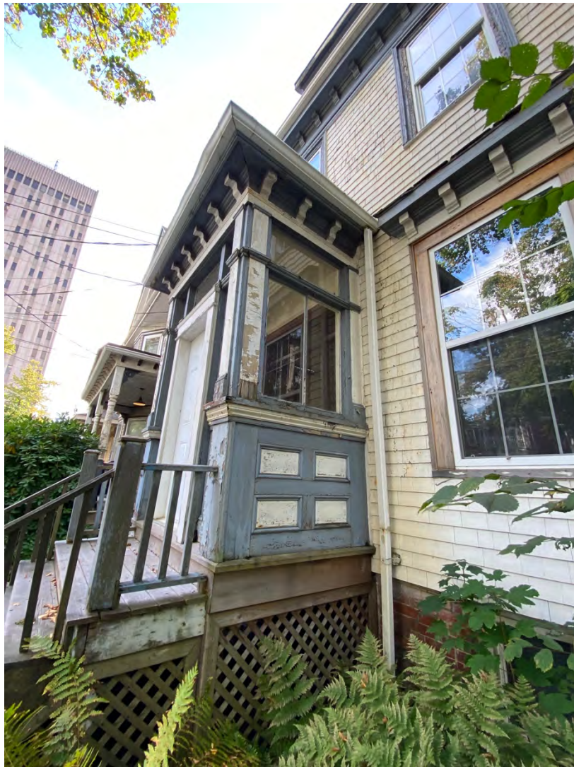
Figure 72g: Tupper Residence, 1468 Carlton Street – porch details
