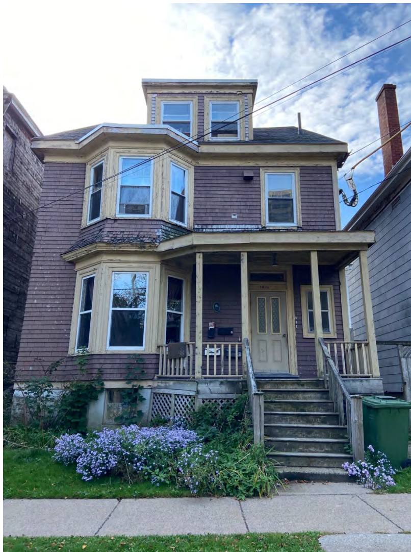
Figure 70a: Neal Residence, 1460 Carlton Street (Front)
