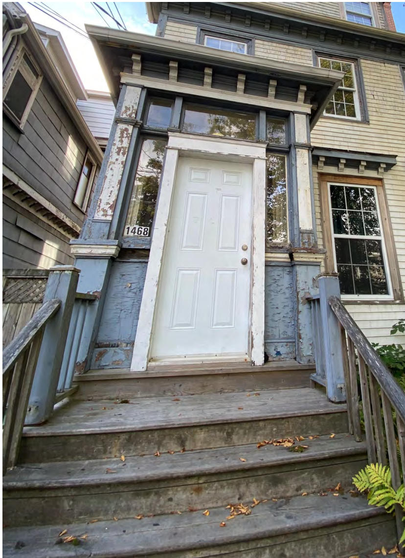
Figure 64: Original porch elements and the modern door enclosure
