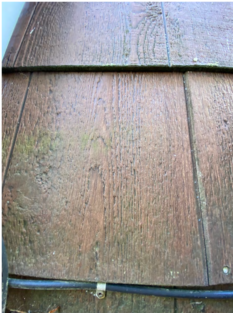
Figure 47: Shingle pattern details, north side
