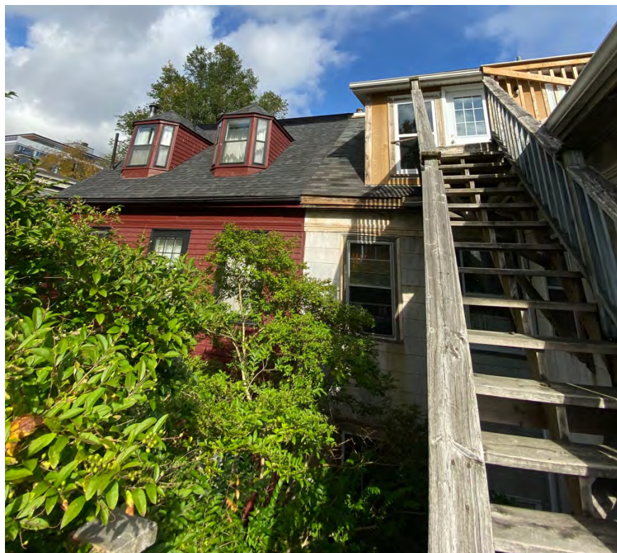
Figure 65: Contrast between the attic of 1474 Carlton Street (left), featuring original Scottish dormers, and 1468 Carlton (right) which has a full width shed dormer
