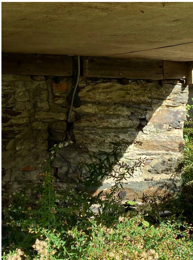
Figure 70e: Neal Residence, 1460 Carlton Street – stone foundation
