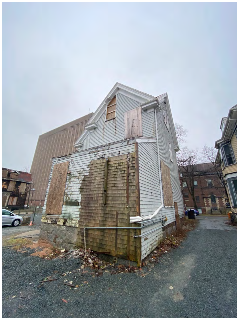
Figure 24b: Shed roof addition at the rear of 5963 College Street
