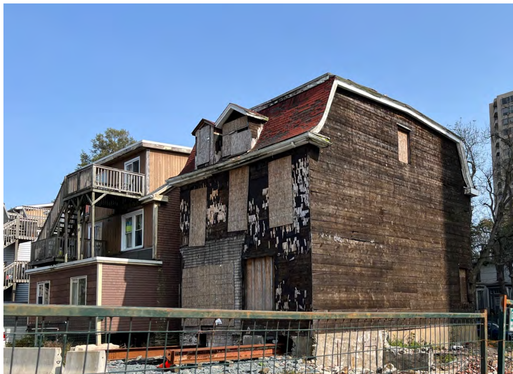
Figure 69b: Crosskill Residence, 1456 Carlton Street (South side and rear)
