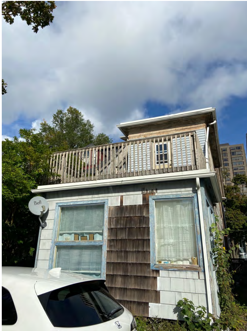
Figure 63b: Tupper Residence, 1468 Carlton Street, rear – south half with later one-storey extension
