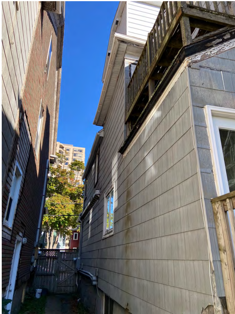
Figure 54d: Keith Residence, 1466 Carlton Street, north side (seen from rear)
