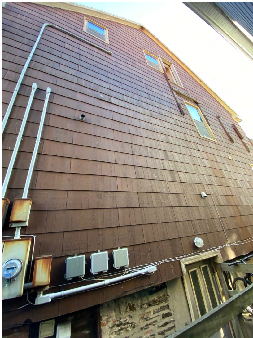
Figure 44c: North side of 1460 Carlton Street
