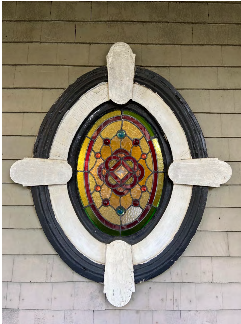
Figure 71g: Keith Residence, 1466 Carlton Street – front oriel window detail
