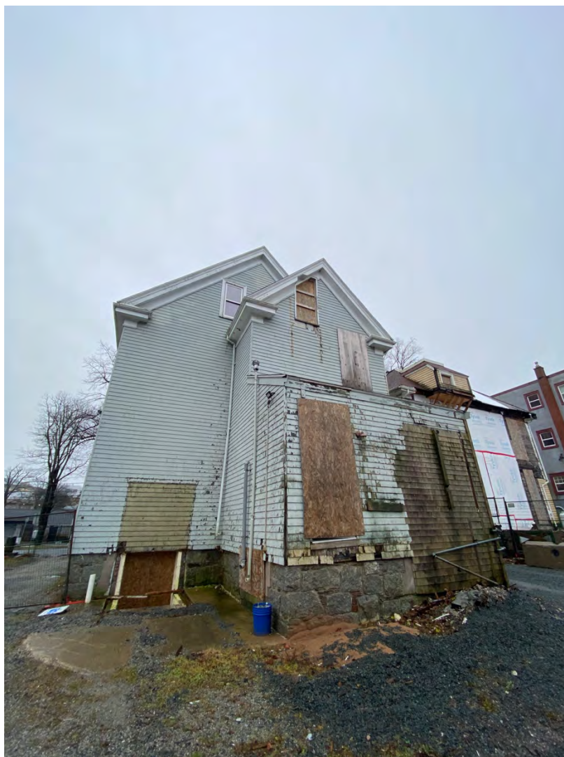
Figure 22c: Rear of 5963 College Street
