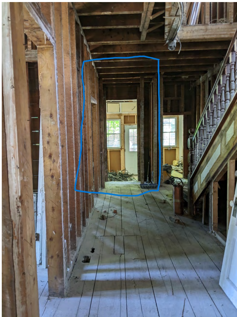
Figure 22d: Interior view of front door and window openings behind enclosed porch, 5963 College Street
