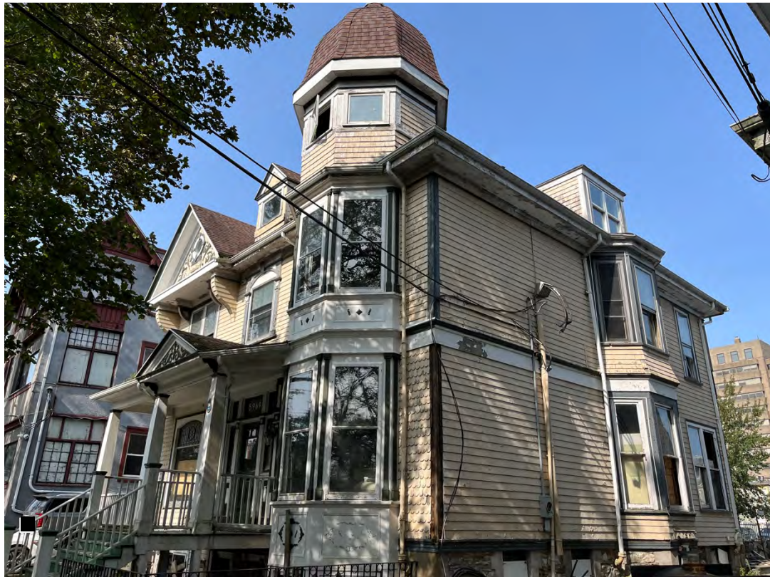
Figure 28b: Gold Cure Institute, 5969 College Street – front and east side
