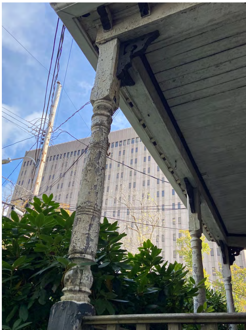
Figure 71f: Keith Residence, 1466 Carlton Street – front porch detail: turned posts, decorative brackets
