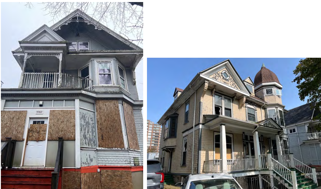
Figures 7e and 7f: 5963 College Street (left) and 5969 College Street (right)
