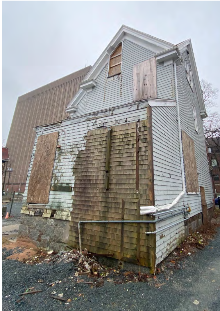
Figure 66d: MacCoy Residence, 5963 College Street (Rear)
