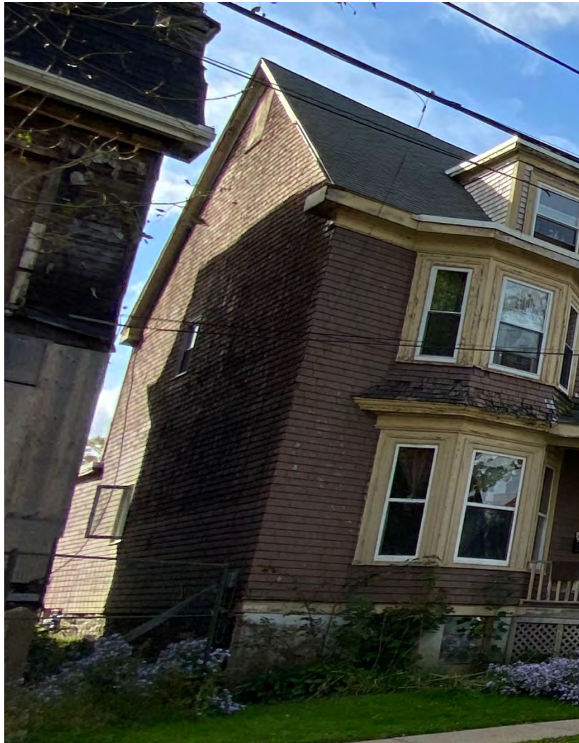
Figure 70c: Neal Residence, 1460 Carlton Street (South side)
