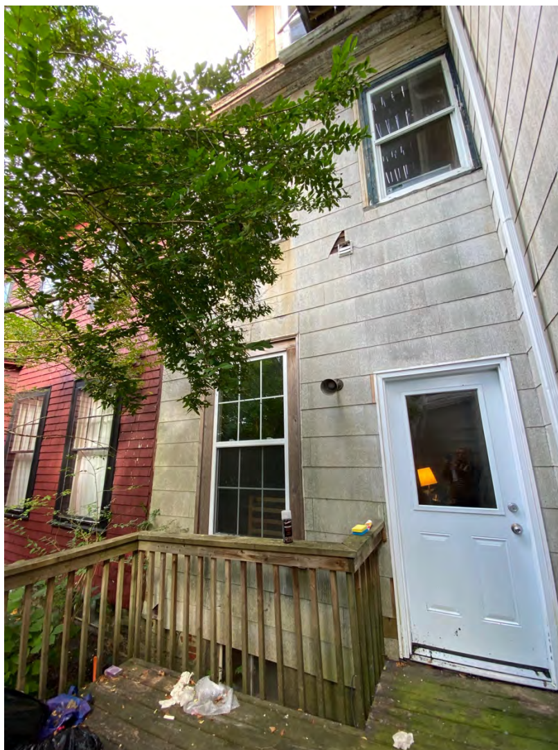
Figure 72b: Tupper Residence, 1468 Carlton Street (Rear face, north half)
