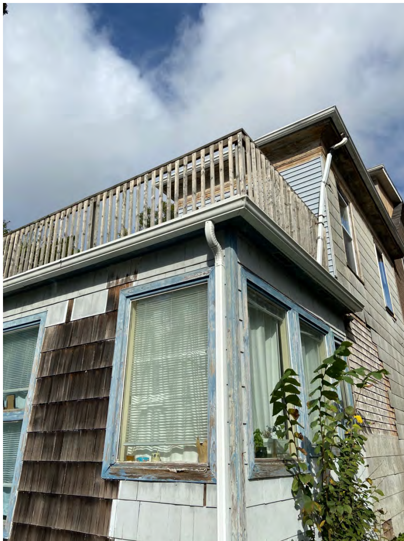
Figure 72c: Tupper Residence, 1468 Carlton Street (Rear, south half)
