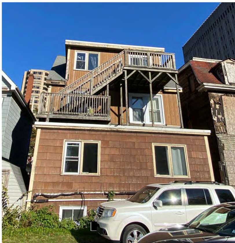
Figure 70b: Neal Residence, 1460 Carlton Street (Rear)
