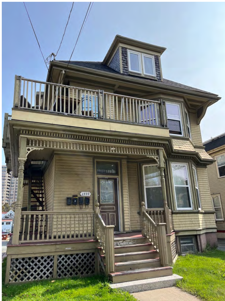
Figure 68a: Mary Belcher Residence, 1377 Robie Street (Front)
