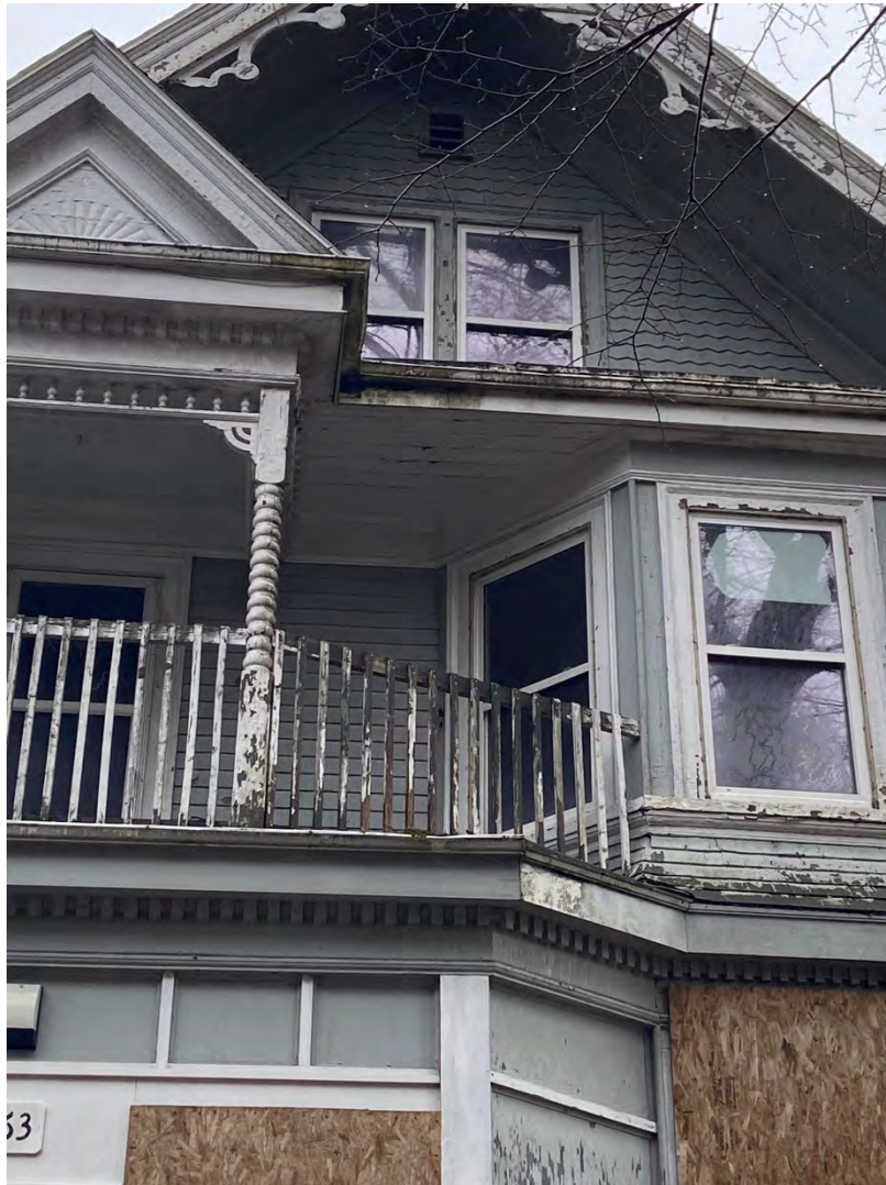
Figure 22b: Upper floor detail of 5963 College Street
