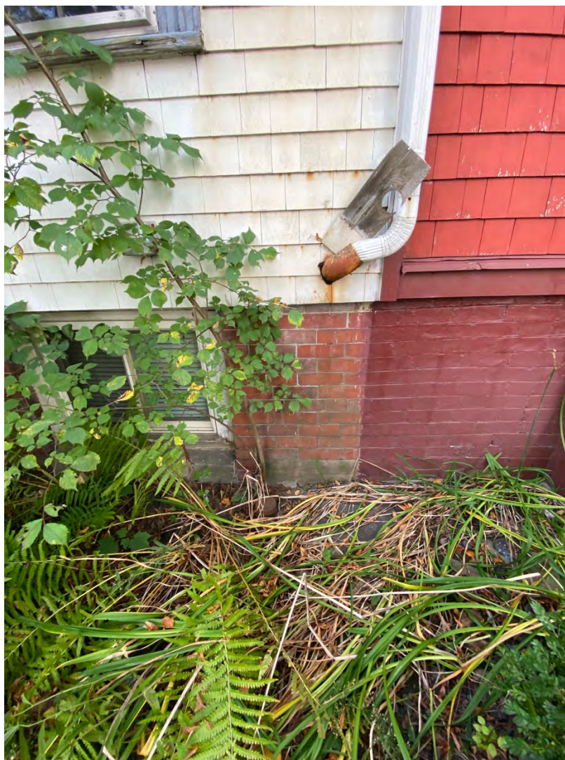
Figure 72f: Tupper Residence, 1468 Carlton Street – brick foundation, front
