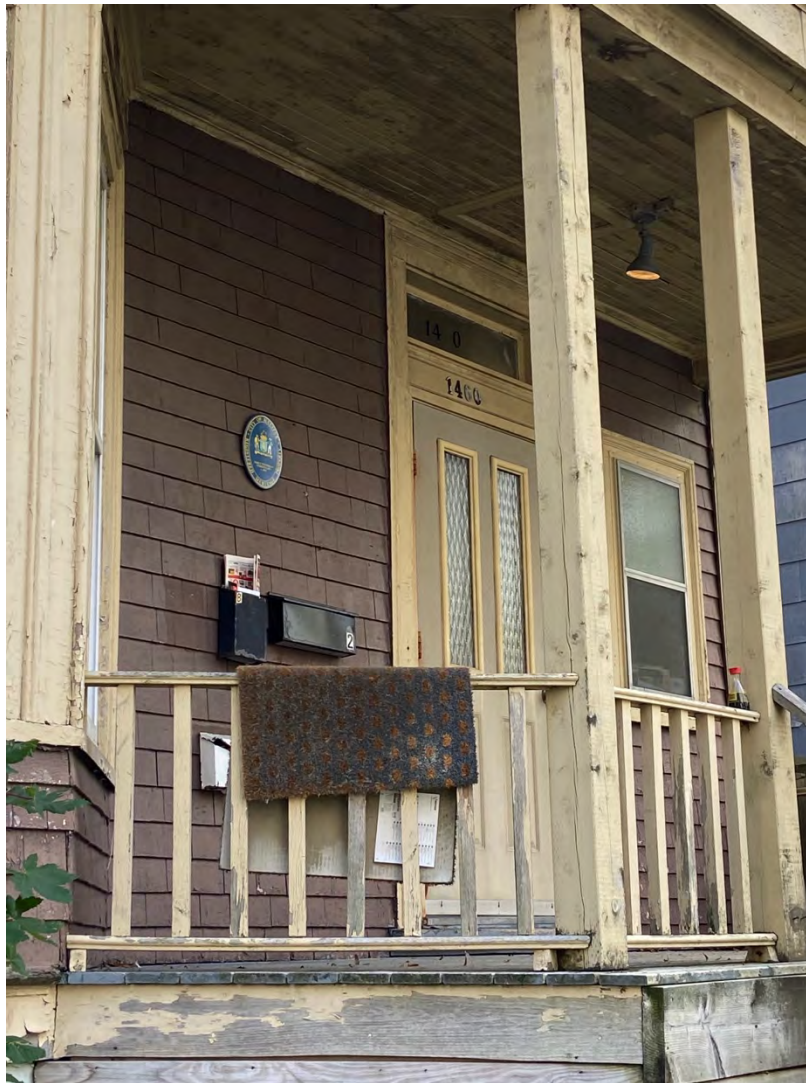
Figure 70g: Neal Residence, 1460 Carlton Street – porch details
