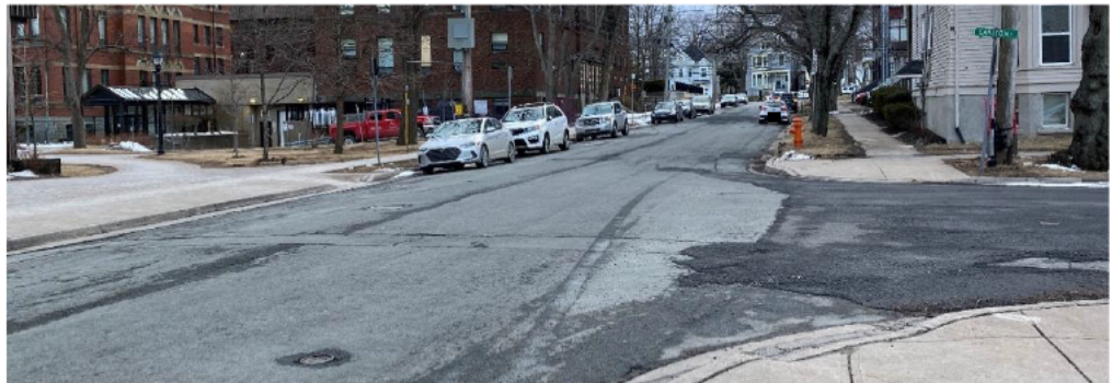
Photo 12 – College Street and Carlton Street
