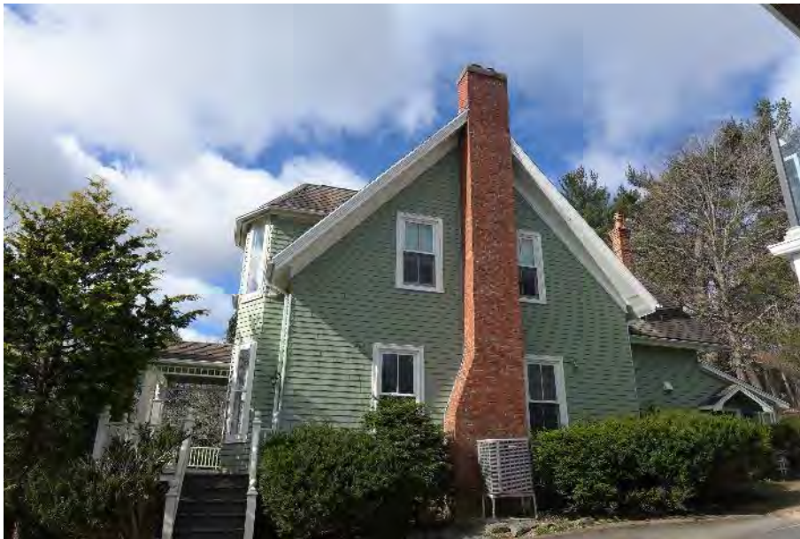
Figure 10: North elevation (Staff photo, April 18, 2024)
