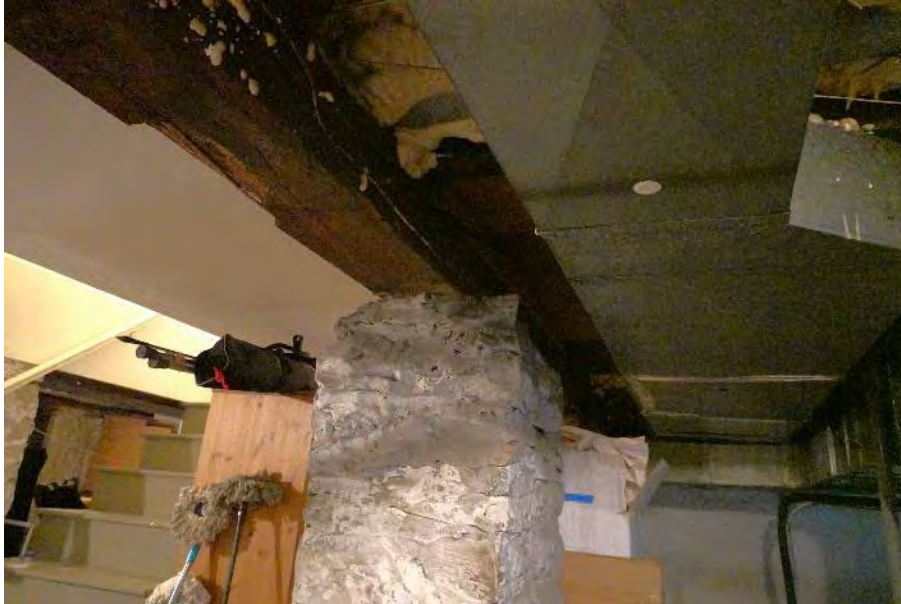
Figure 8: Rock foundation and wood beams as visible in the basement (Staff photo, April 18, 2024)
