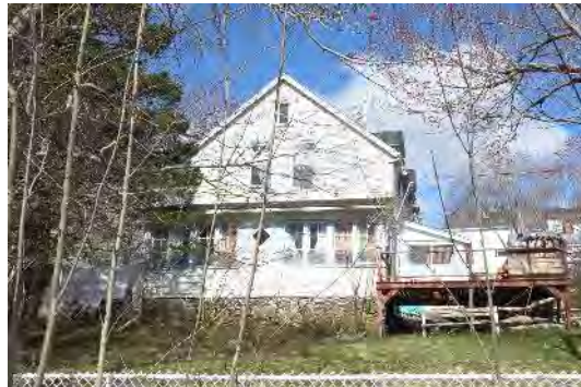
Figure 27: 9 Division Street (Staff photo, April 18, 2024)
