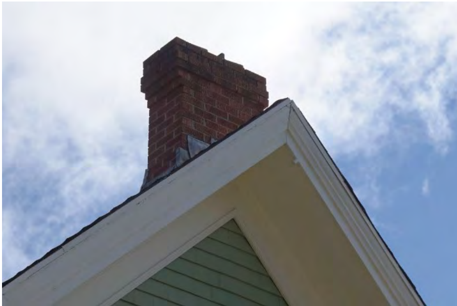
Figure 14: Single-stack brick chimney and moulded fascia and frieze (Staff photo, April 18, 2024)
