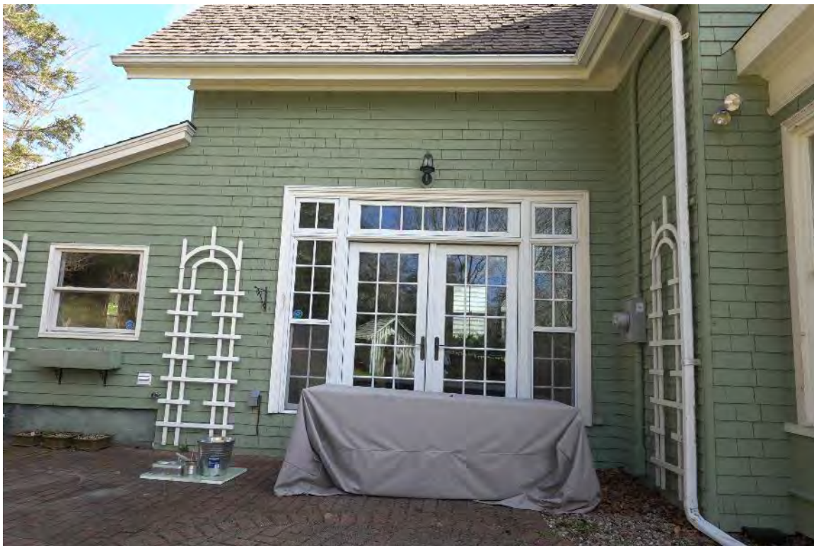
Figure 21: Two French doors with surrounding lights were added to the south side of the rear wing (Staff photo, April 18, 2024)
