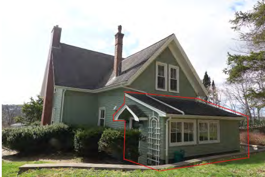
Figure 18: Rear addition highlighted with redlines (Staff photo, April 18, 2024)
