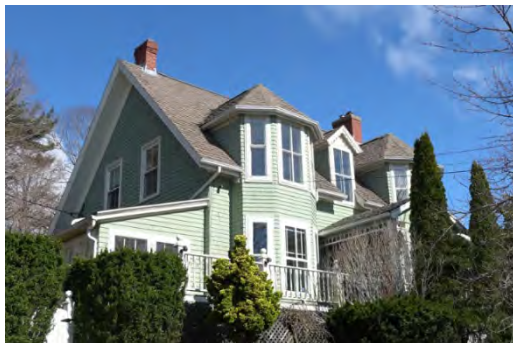
Figure 1: 6 First Avenue, April 2024
