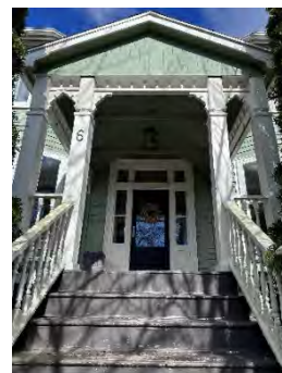
Figure 2: The porch and entry door of the subject building, July 2024
