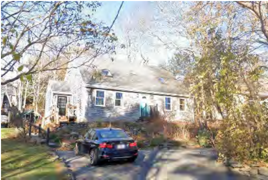
Figure 24: 14 First Avenue (Google Streetview, November, 2022)
