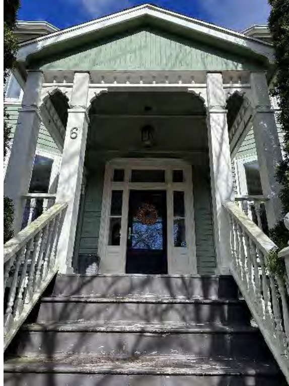
Figure 15: Pedimented porch with fretted railings, bargeboards, brackets, and square posts; Under the porch, the main entry door with side light, transom lights, and decorative panels and trims. (Staff photo, April 18, 2024)
