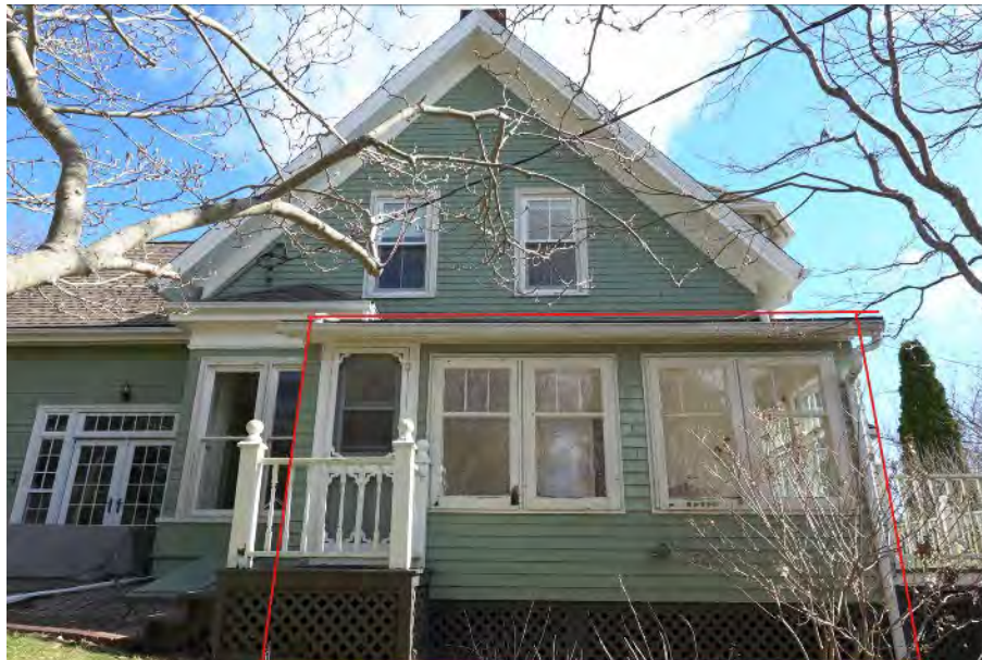
Figure 19: South addition highlighted with redlines, recognized as a character-defining element as an early alteration (Staff photo, April 18, 2024)
