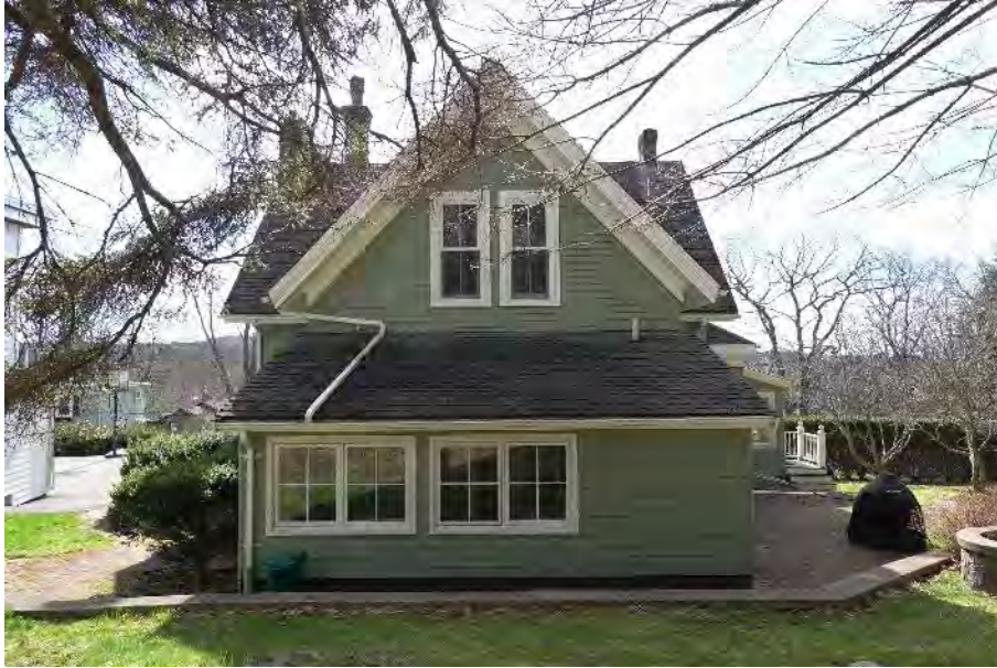
Figure 11: West elevation (Staff photo, April 18, 2024)
