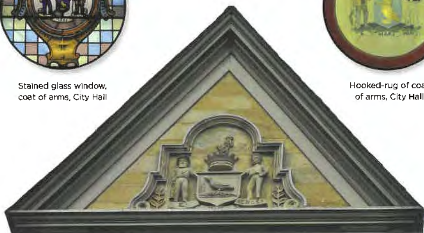
Coat of arms sculpture on City Hall exterior
