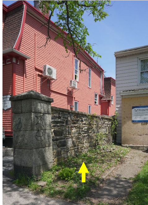
Mid-1800s stone masonry wall (May 31, 2023)
