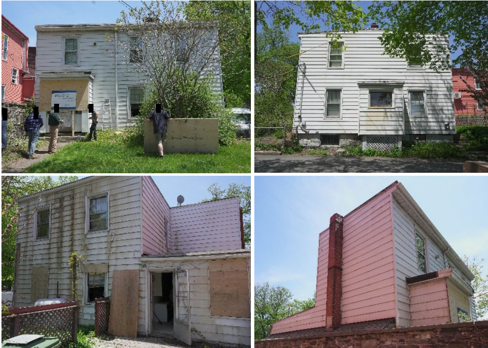
Elevation photos taken during site visit (May 31, 2023)
