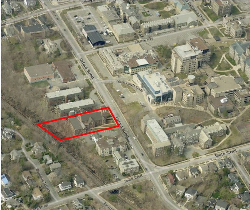
Surrounding area of the subject building
