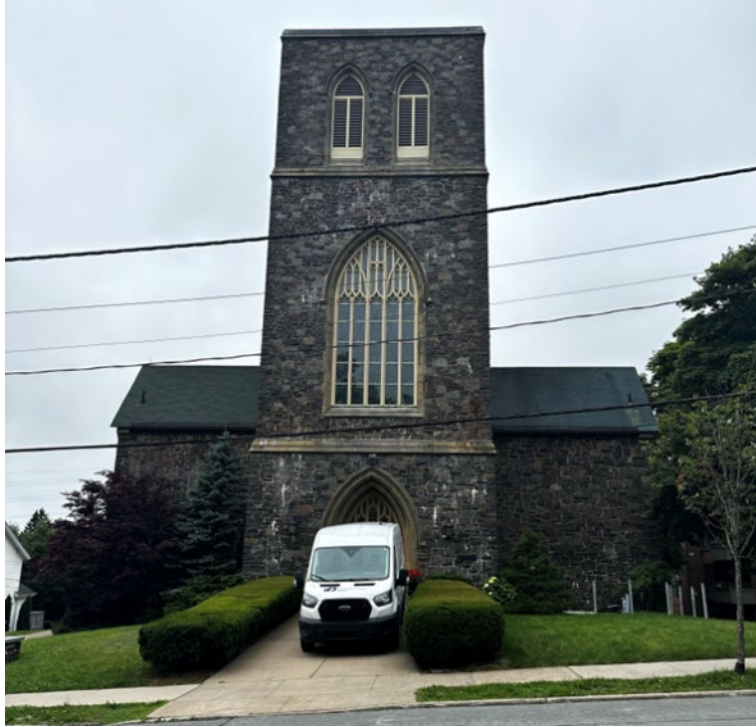
Figure 22: East elevation (July 17, 2024)
