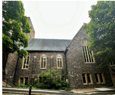
Figure 3: North elevation, July 2024
