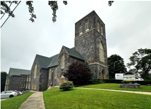
Figure 2: South and east elevations, July 2024
