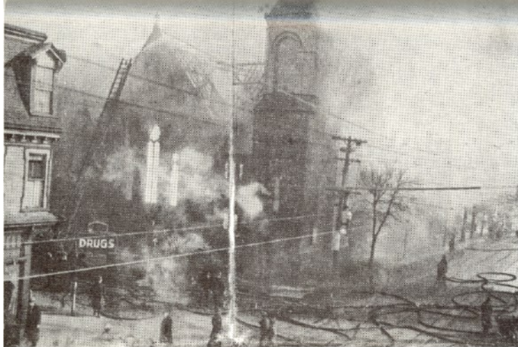
Figure 8: Spring Garden Road First Baptist Church during the fire, March 21, 1942 1,4
