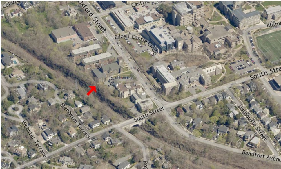
Figure 28: The subject building denoted by a red arrow and the surrounding area, 2024
