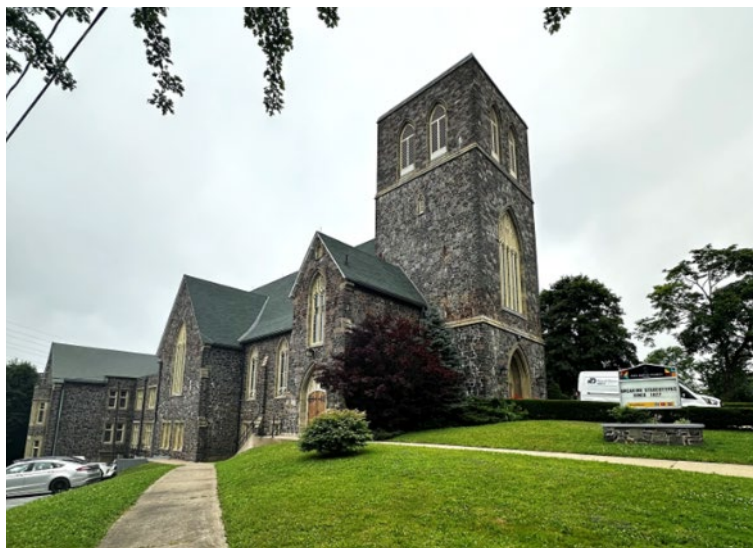
Figure 21: South and east elevations (July 17, 2024)
