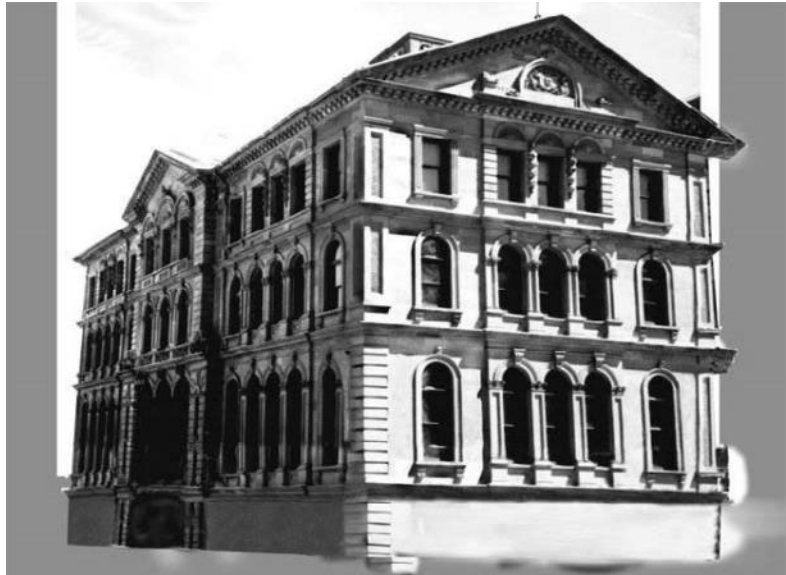
Figure 13: Old Post Office (Art Gallery of Nova Scotia), one of the representative projects of Brookfield Construction Company
