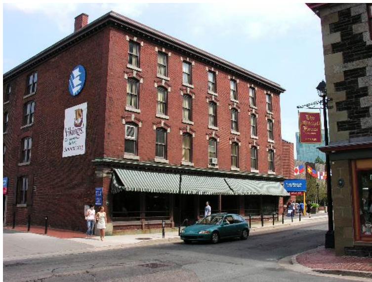
Figure 11: Dr. Allan Duffus led the Robertson Hardware Building restoration project, which became part of the Maritime Museum complex. Photo taken in 2009.
