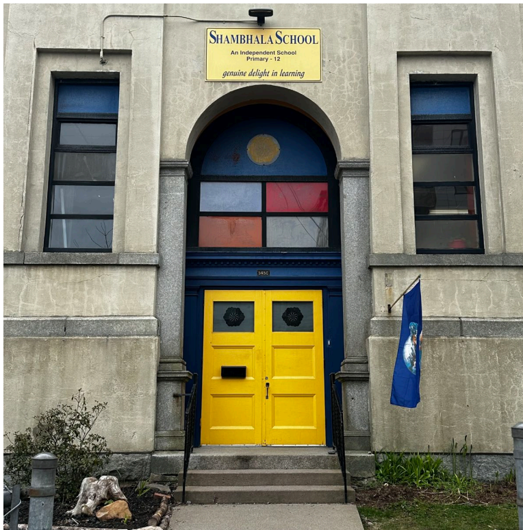
Figure 20: Double-leaf, wood and glazed entrance on the north elevation with multiple-light flat transom and shaped transom above, and granite columns with plinths (May 1, 2024)
