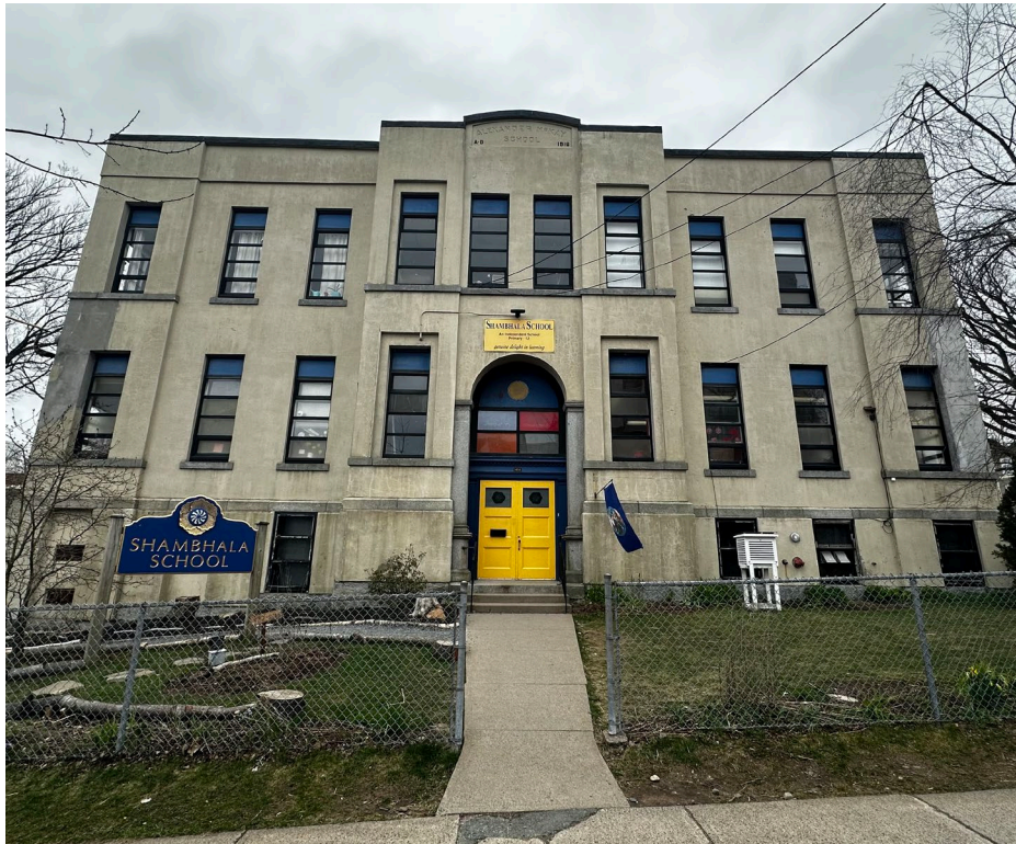
Figure 13: North elevation of the original portion of 5450 Russell Street (May 1, 2024)
