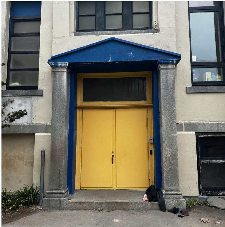
Figure 21: West Elevation double-leaf wood entrance with flat transom and granite piers (May 1, 2024)
