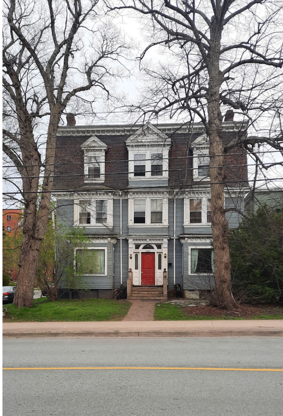
Figure 15: North (Inglis) façade of 5492 Inglis Street (May 4, 2021)
