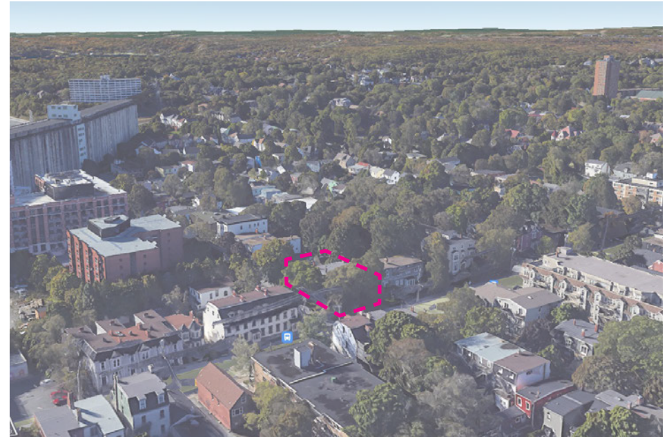
AERIAL VIEW LOOKING TOWARDS INGLIS AND SOUTH BLAND STREETS
