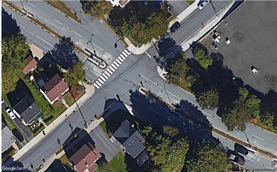
Figure 5: Intersection of Young Street at Devonshire Avenue
