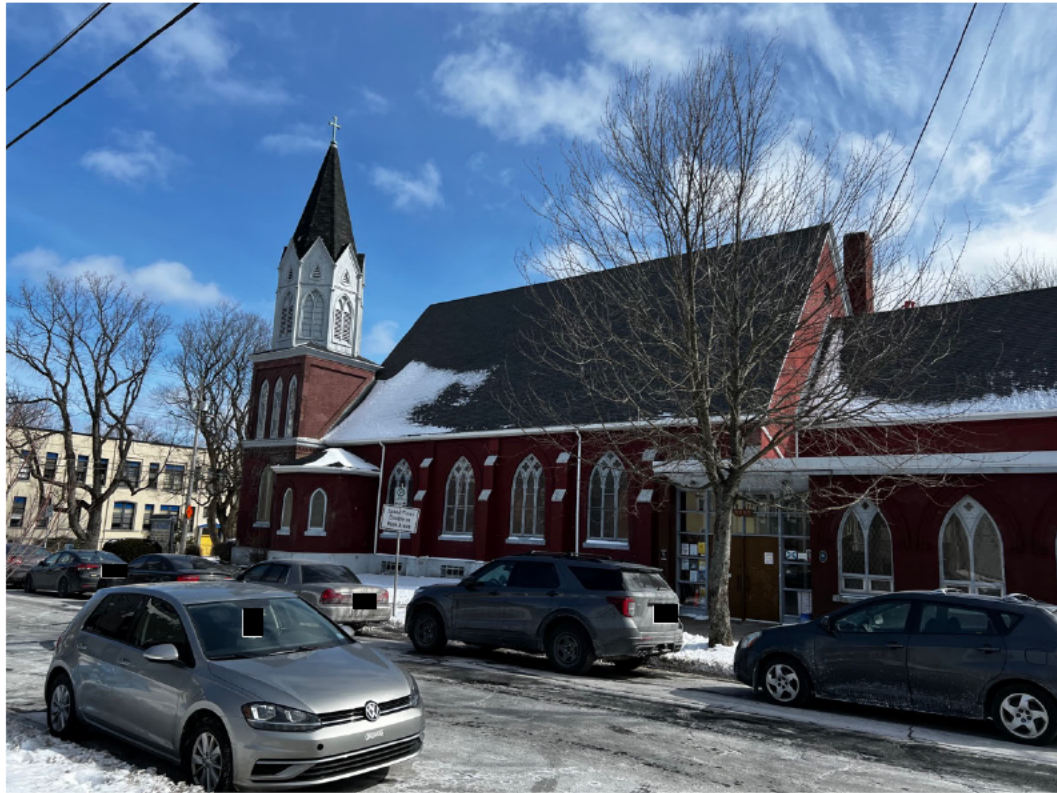
Figure 29b: Context of St. Mark's Church, 5522 Russell Street (seen from side, along Russell Street)
