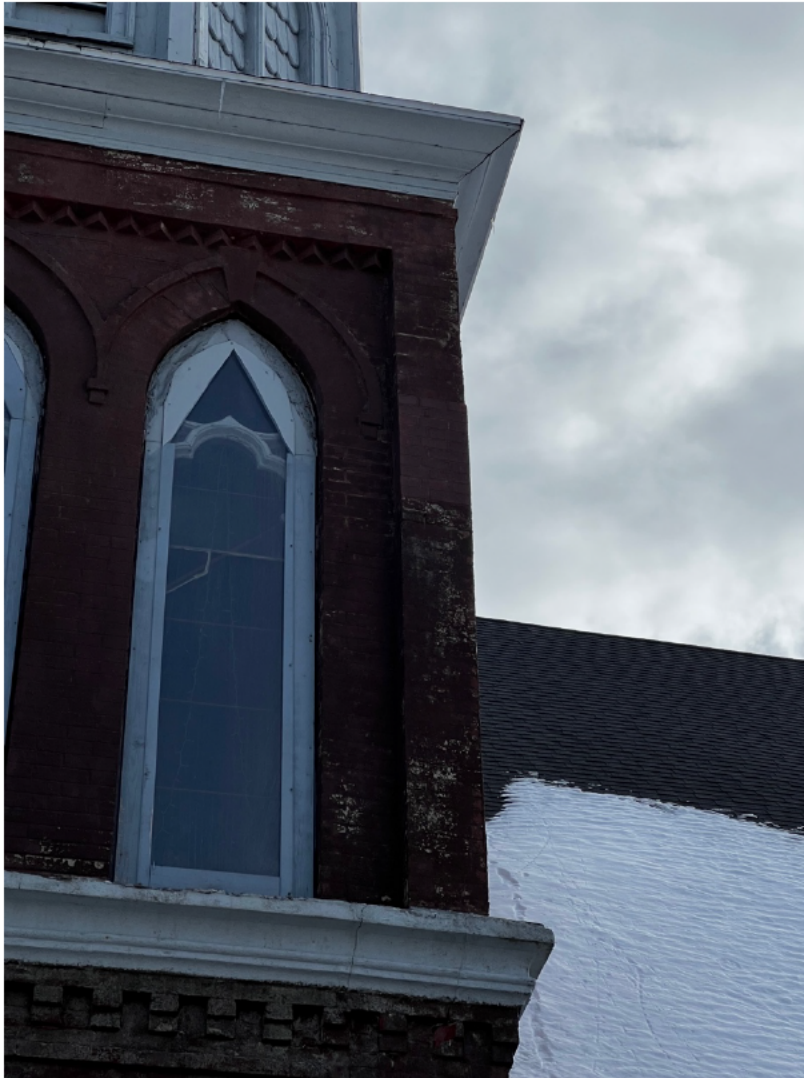
Figure 41i: St. Mark's Church, 5522 Russell Street (upper side section of north tower)
