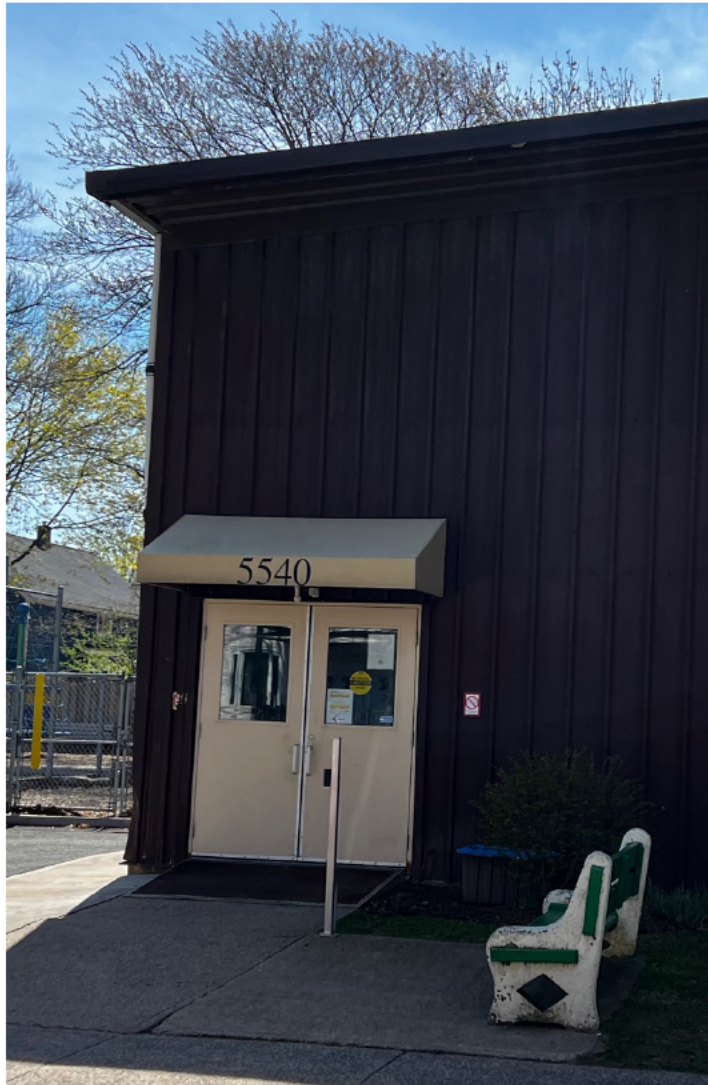
Figure 40: Paired entry doors, 5540 Russell Street
