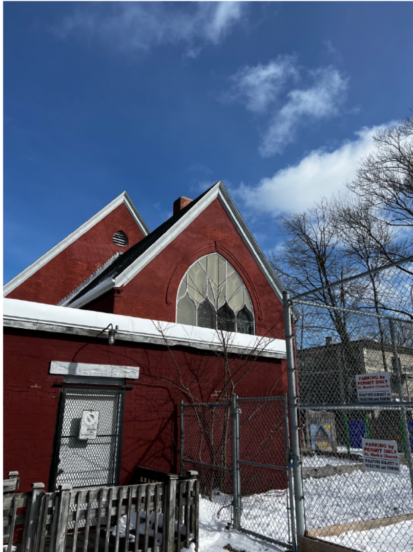
Figure 31c: Single-storey addition wrapping around the west side of 5522 Russell Street, with a single emergency exit door
