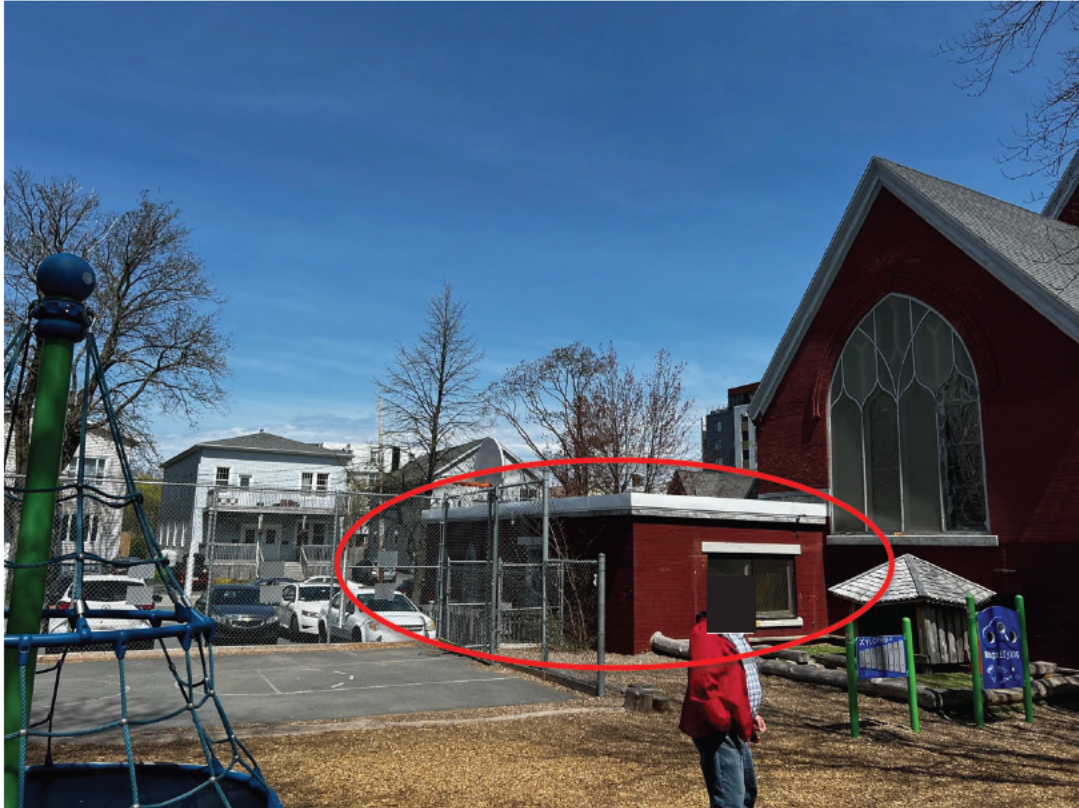
Figure 31b: Single-storey addition on the north side of 5522 Russell Street, seen from the rear and ending at the edge of the apse windows (circled)
