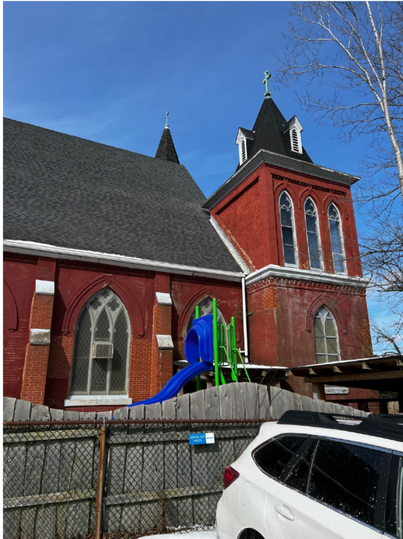
Figure 41b: St. Mark's Church, 5522 Russell Street (south side and south tower)
