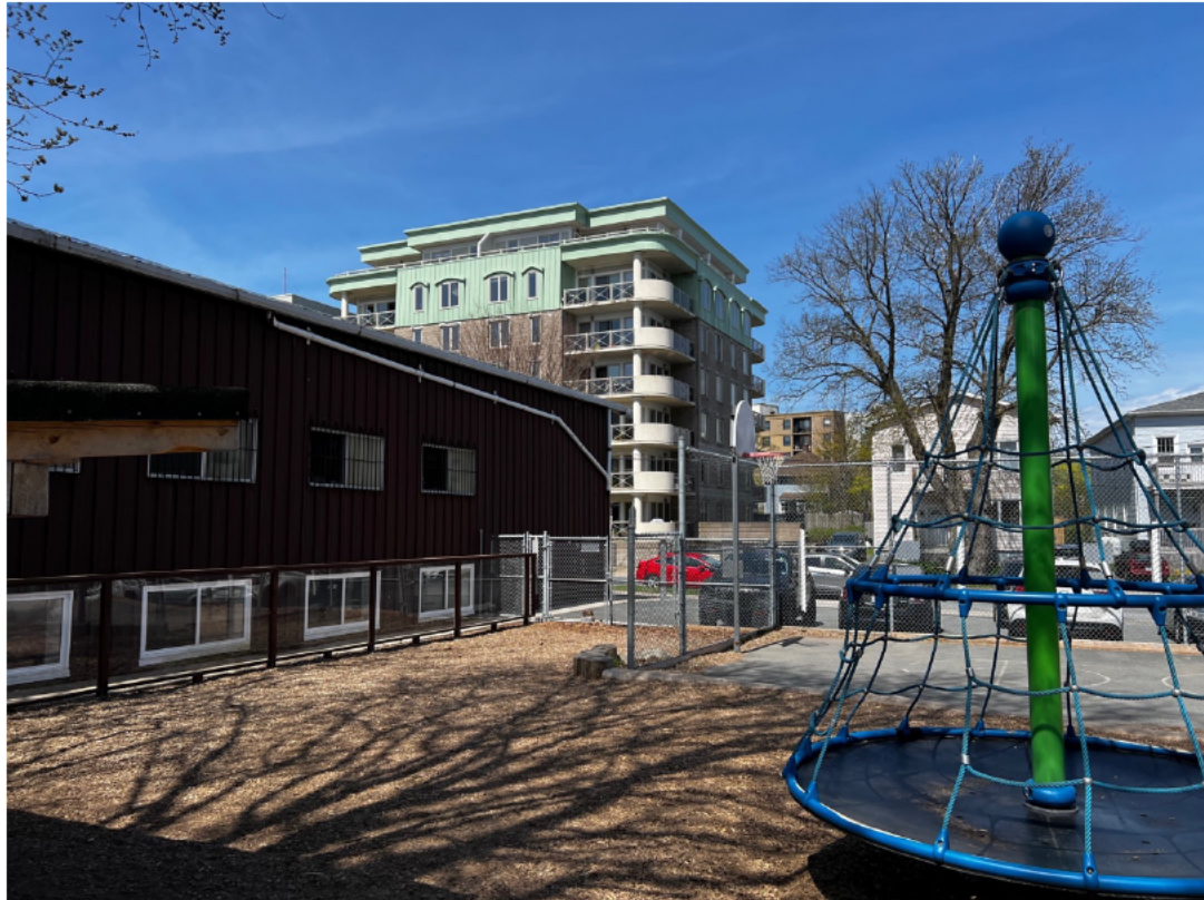
Figure 39a: 5540 Russell Street – east side and open space between church
