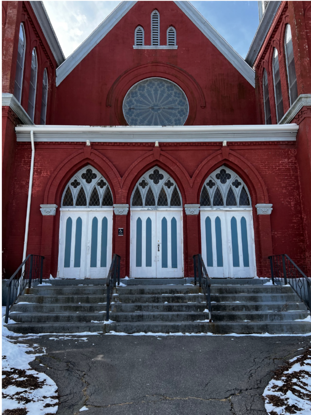
Figure 30a: Front entry of 5522 Russell Street with flanking towers
