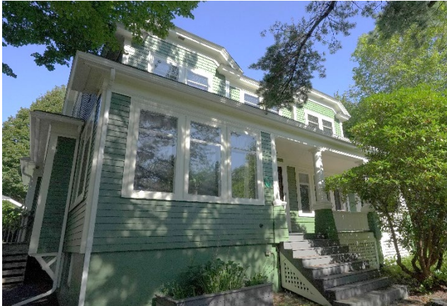
Existing heritage building
