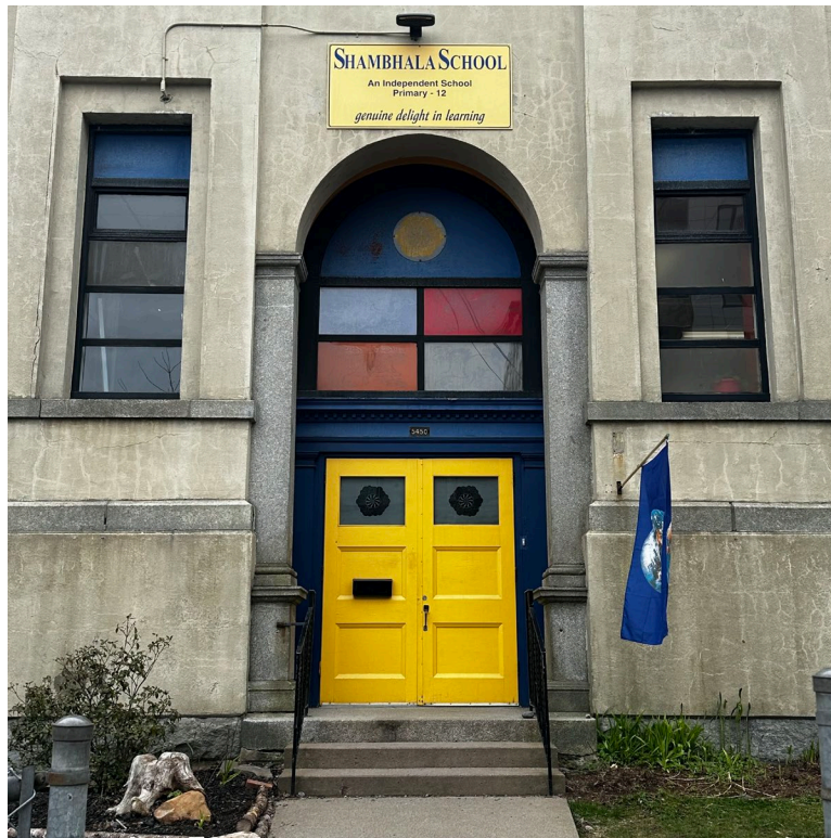
Figure 20: Double-leaf, wood and glazed entrance on the north elevation with multiple-light flat transom and shaped transom above, and granite columns with plinths (May 1, 2024)
