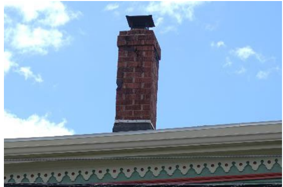
Figure 16: Brick Chimney (April 26, 2024)
