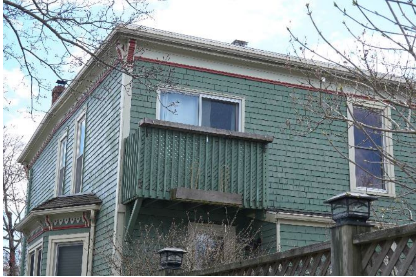
Figure 20: Added Balcony At The Rear (April 26, 2024)
