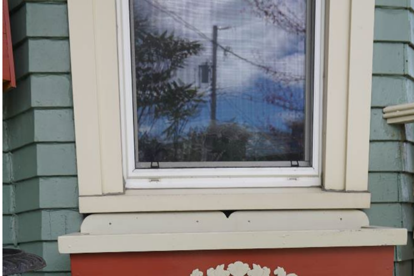
Figure 18: The sashes have been replaced with vinyl, and frame has metal cladding (April 26, 2024)
