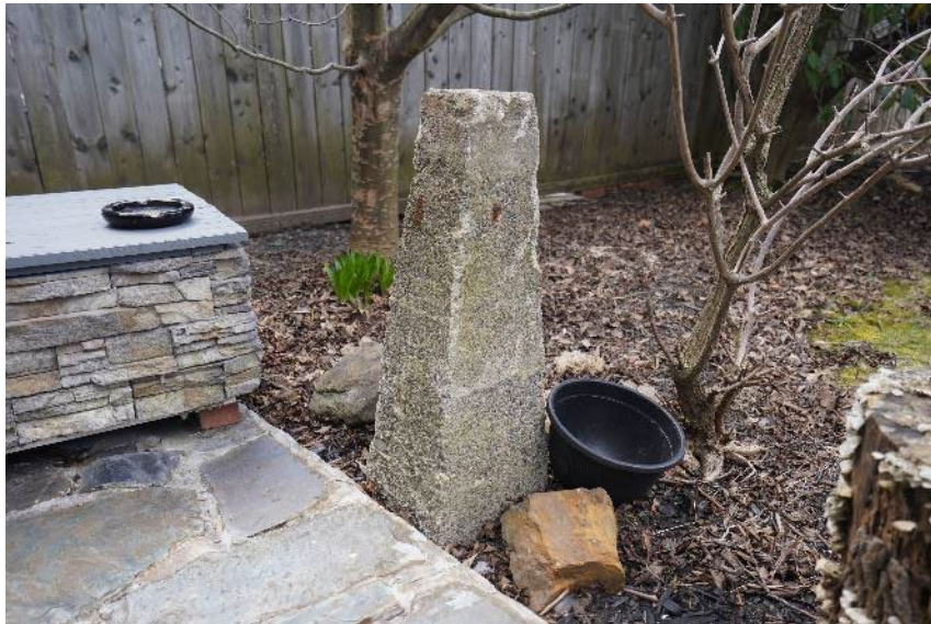
Figure 29: The Removed Support Concrete Post For The Rear Addition (April 26, 2024)
