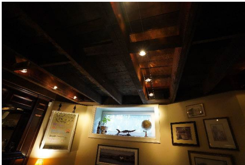
Figure 6: Structural elements in the basement of the subject property (April 26, 2024)
