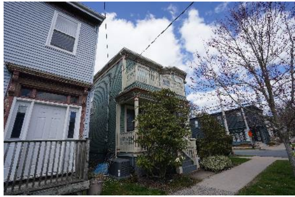
Figure 10: West Elevation (April 26, 2024)
