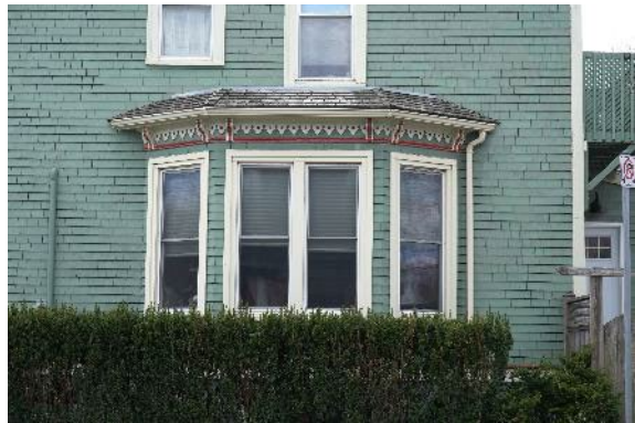
Figure 12: One-storey bay window on the east elevation with three one-over-one wood-framed windows with running trims and corbel detailing (April 26, 2024)
