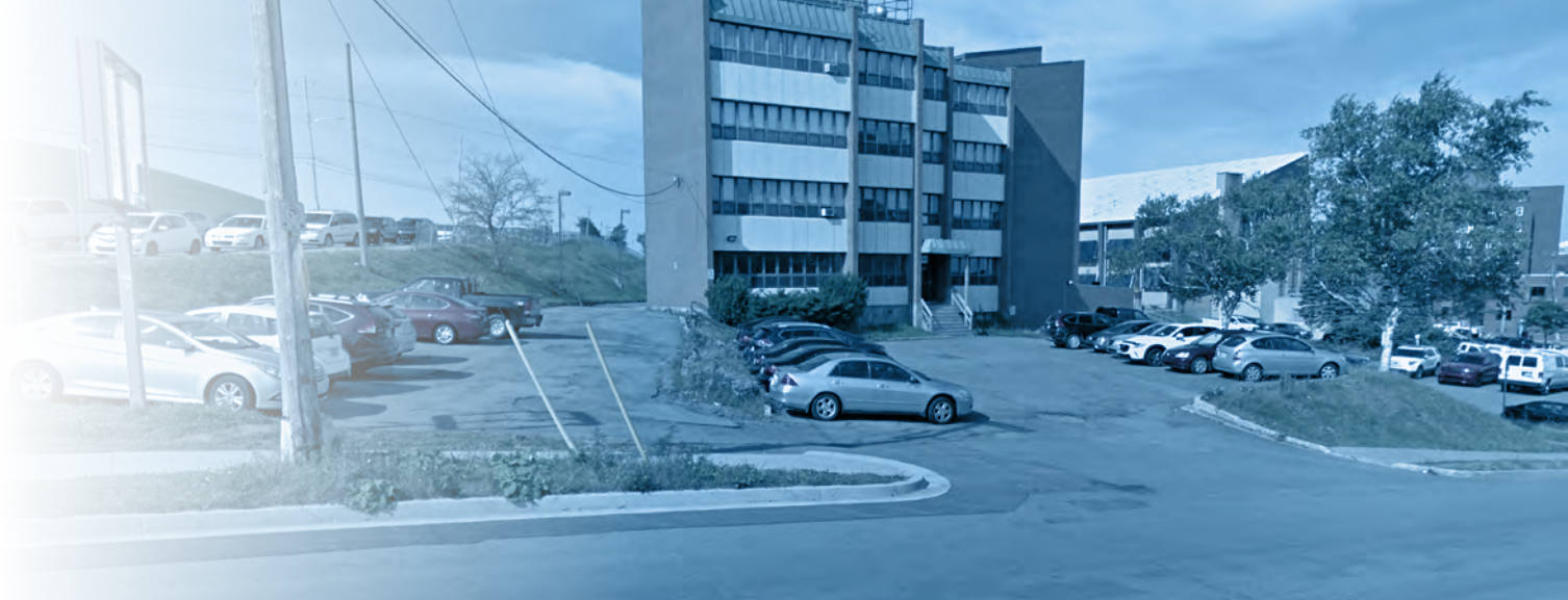
FIGURE 2. CANADIAN BLOOD SERVICES BUILDING Scheduled for 2022 Demolition
