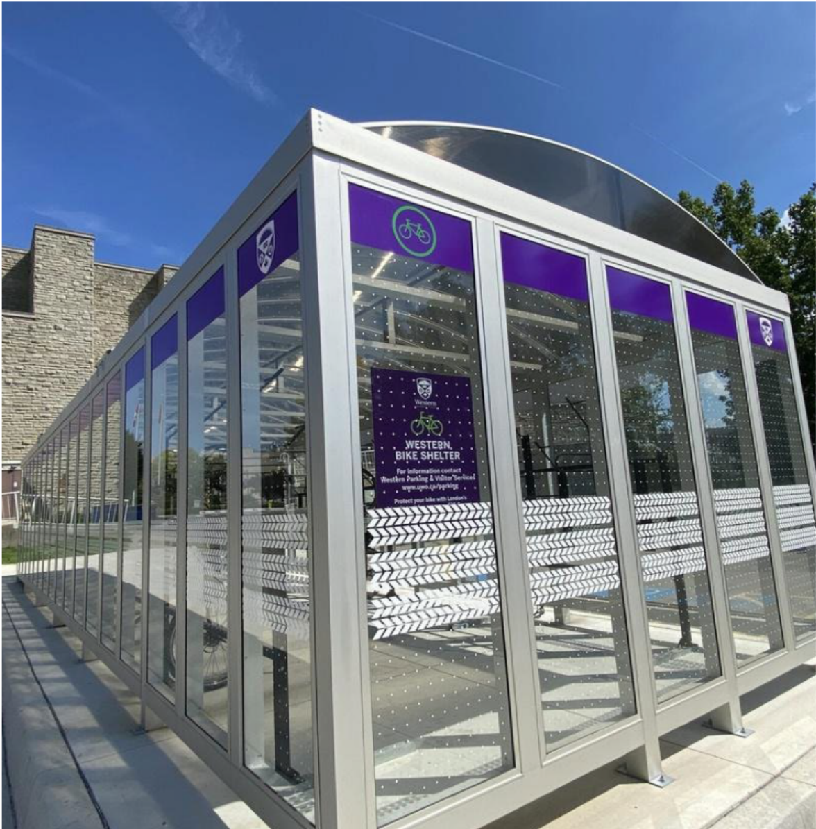
Bird friendly retrofit of Alumni Hall bike storage shelter at Western University. Photo: Brendon Samuels
