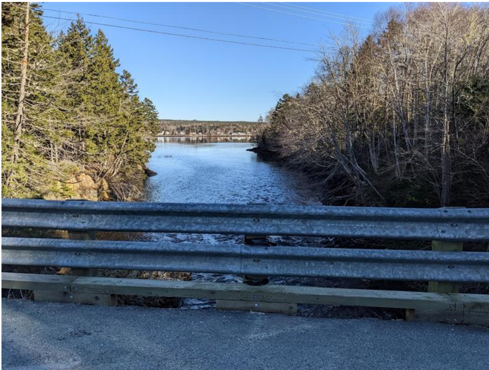
Figure 11-8: Deployment location at West Side Road bridge, facing towards Sheet Harbour. The instrument can be seen attached to the central guardrail post.
