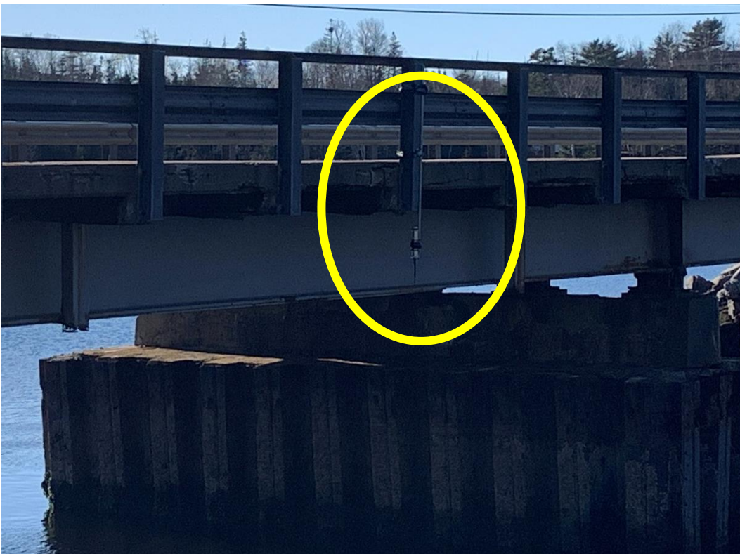
Figure 11-12: The deployed instrument, seen hanging below a guardrail post above Jeddore Harbour.
