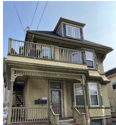
Mary Belcher Building (west elevation)
