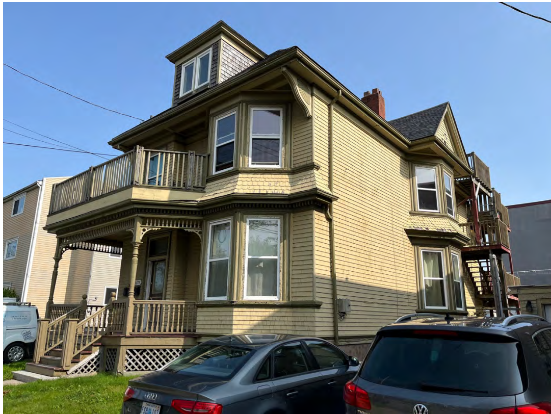
Figure 29a: 1377 Robie Street, front and south side
