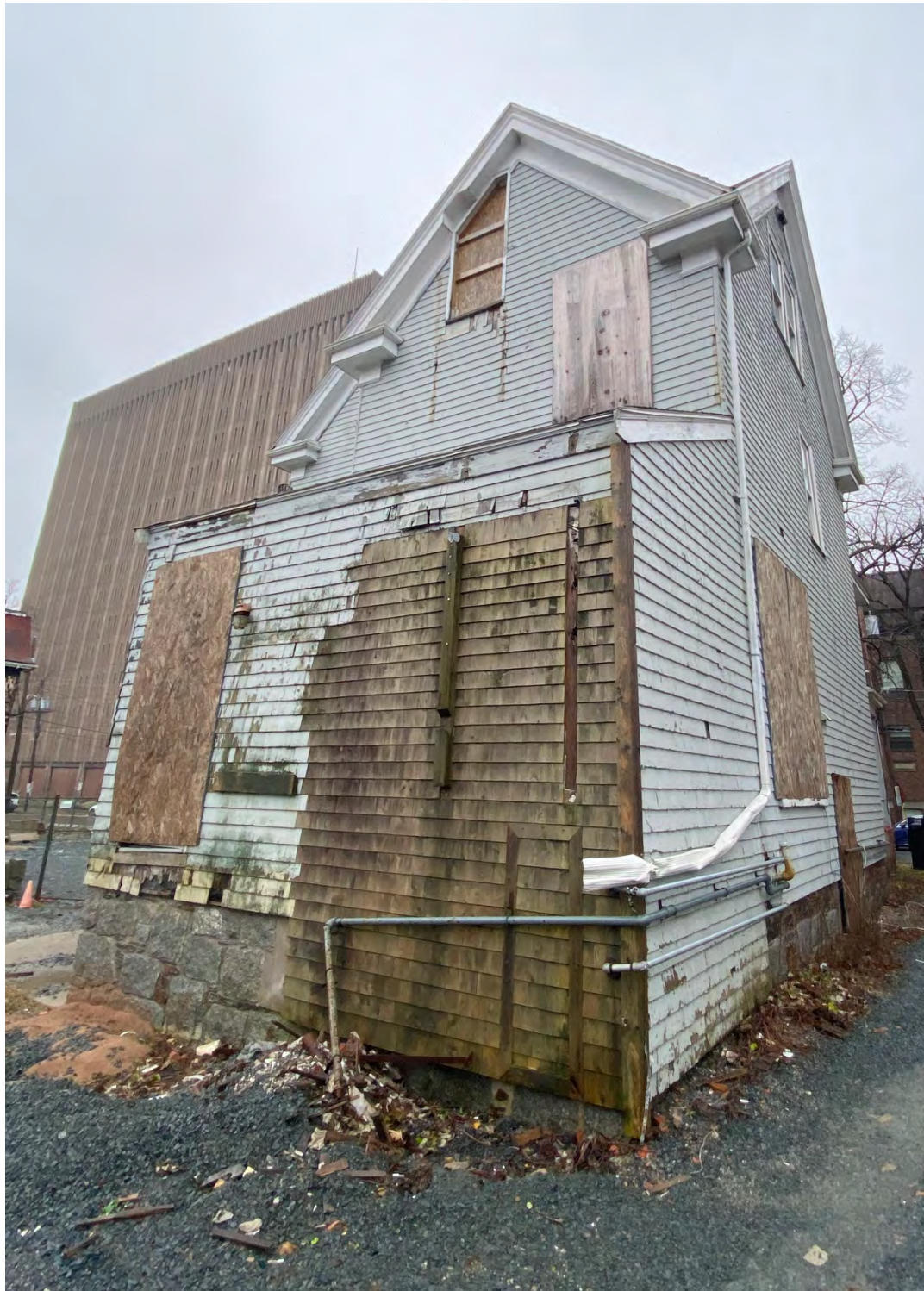
Figure 35d: MacCoy Residence, 5963 College Street (Rear)
