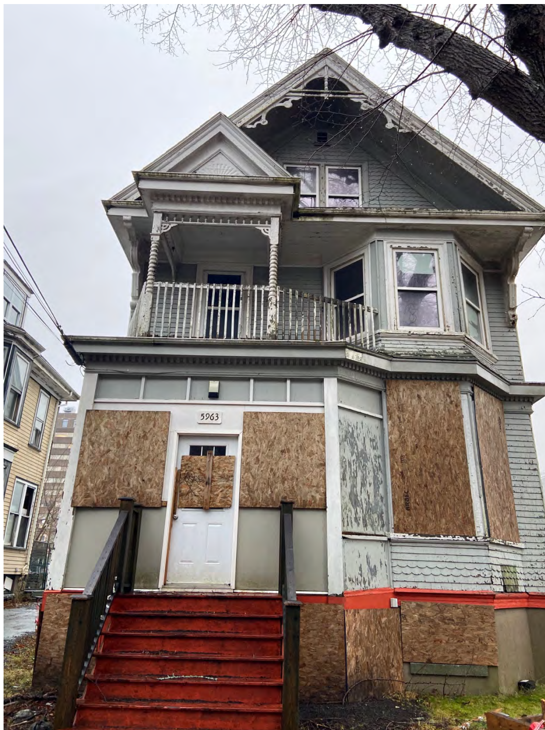
Figure 35a: MacCoy Residence, 5963 College Street (Front)
