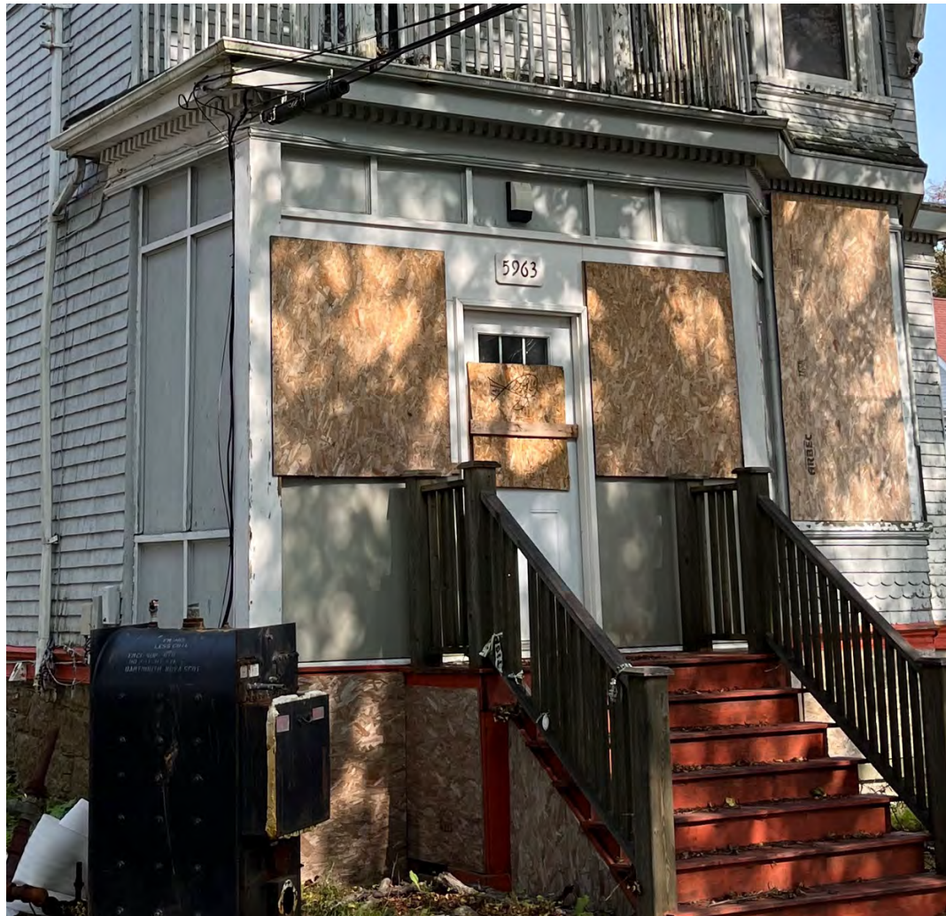
Figure 23a: Front porch enclosure of 5963 College Street
