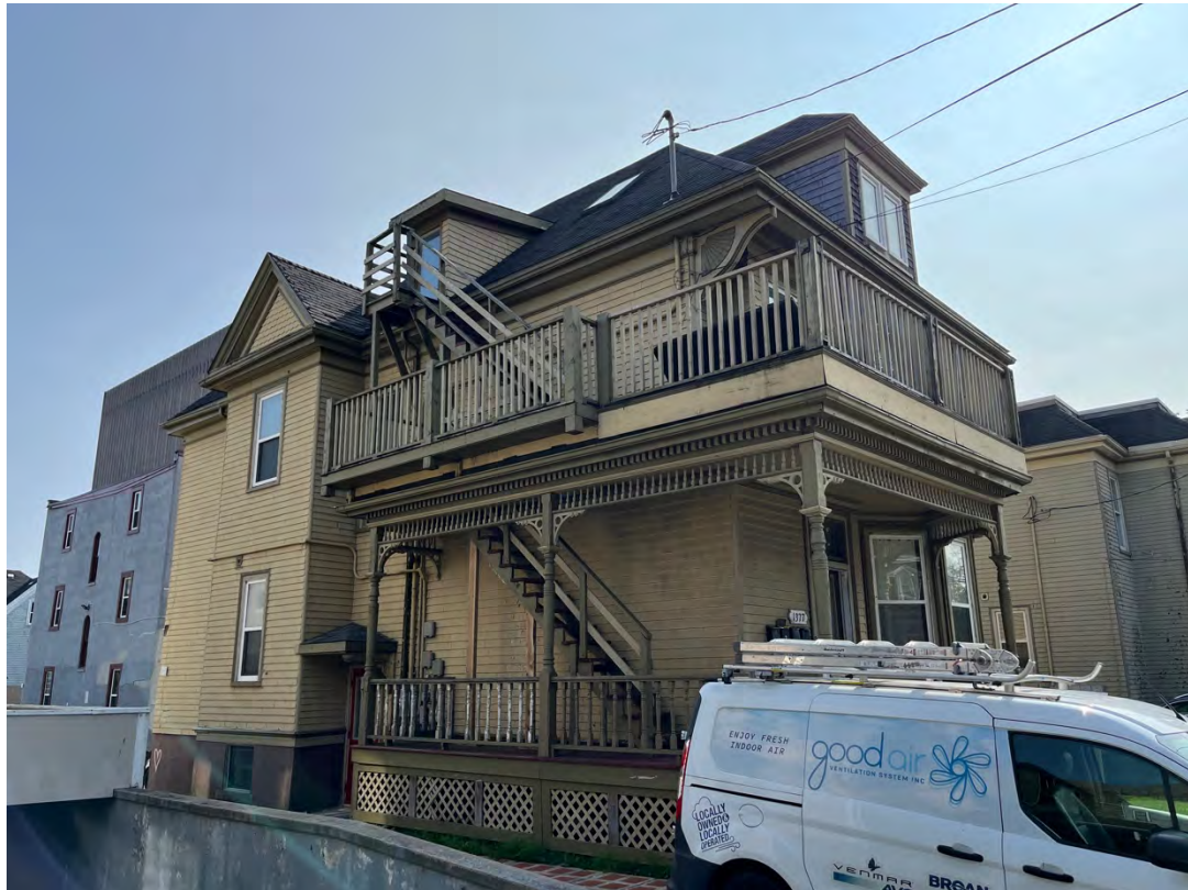
Figure 29b: 1377 Robie Street, front and north side
