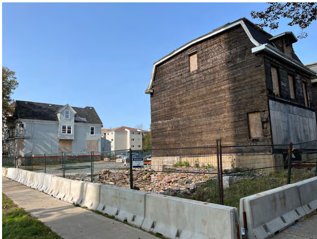
Figure 32: Corner of Carlton and College Street – vacant site following the collapse of the house previously located here
