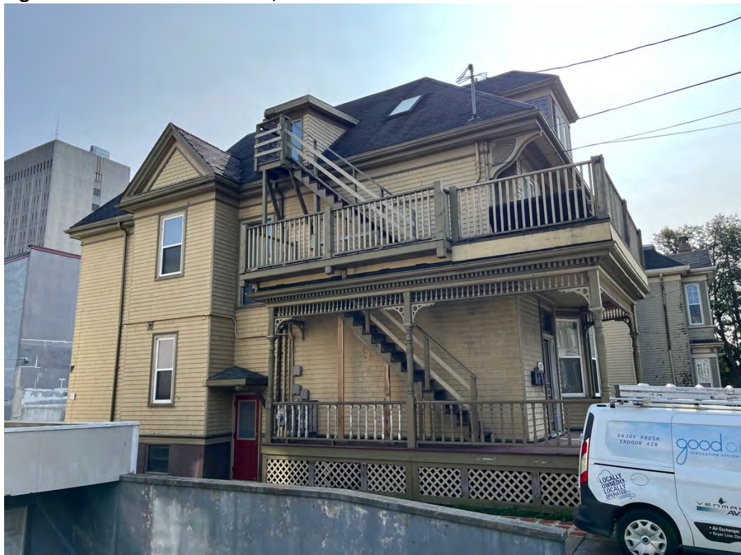
Figure 29c: 1377 Robie Street, north side with wrap-around porch
