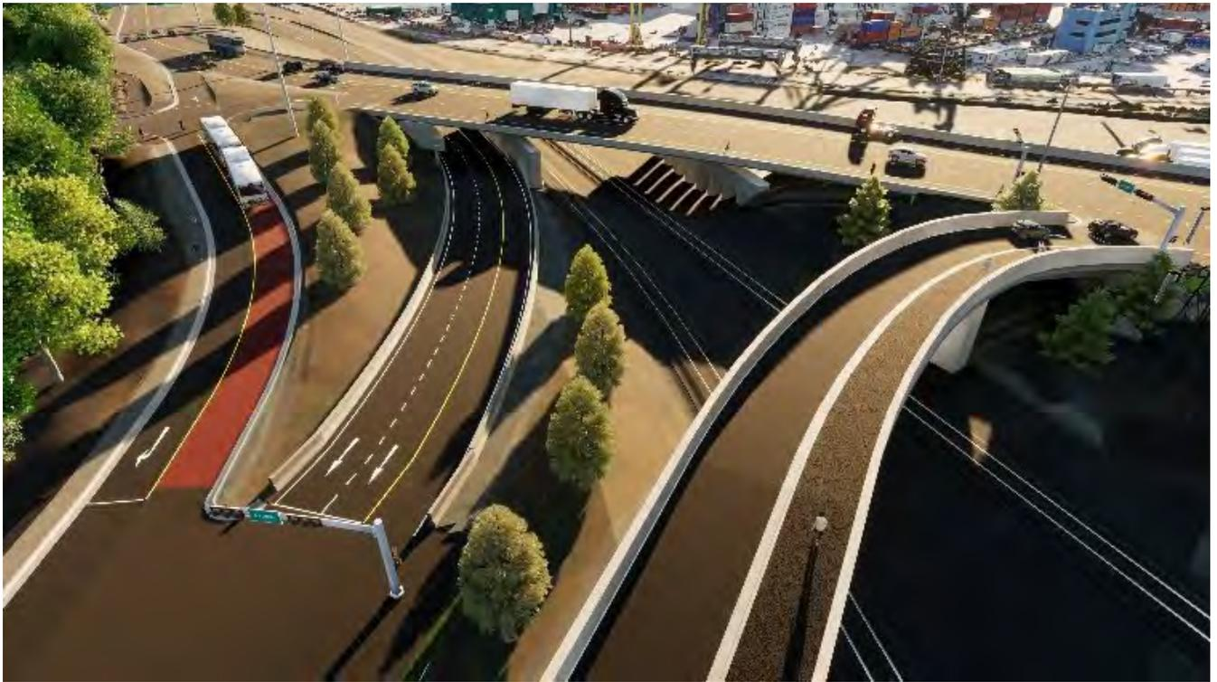
Figure 1-8: Joseph Howe Displaced Left Turn and DVK Ramp Signal and Multi-Use Path
