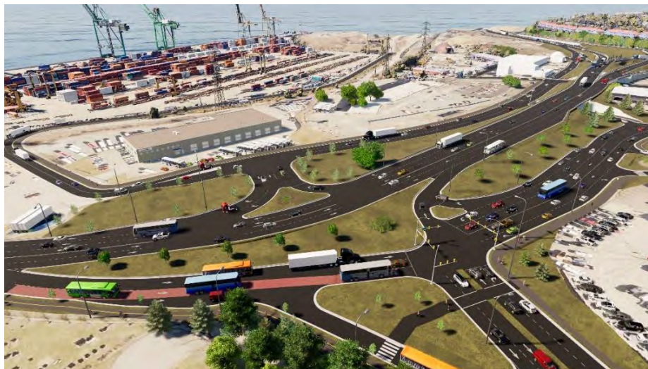
Figure 1 Aerial View of the Reconfigured Windsor Street Exchange
