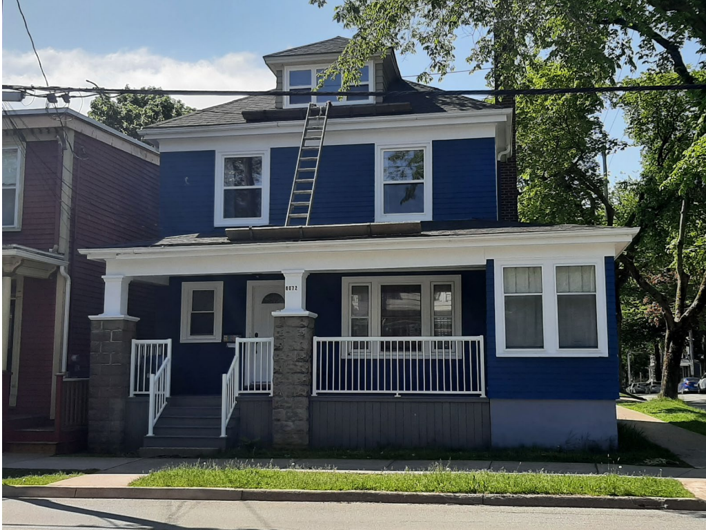
Figure 15: Concrete block veranda posts at 6072 Jubilee Road (Staff Photo, June 16, 2023)
