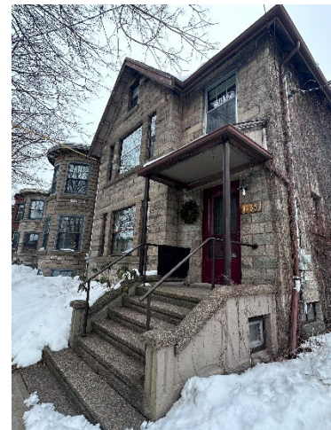
Figure 2: West elevation of 1735 Henry Street (Staff photo, February 16, 2024)
