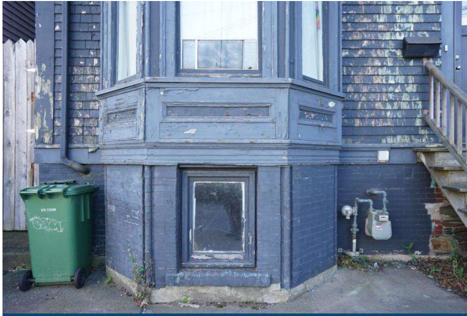
Above: Close-up of stone and brick foundation
