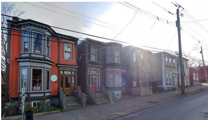
Late Victorian streetscape on North Street (November, 2022).
