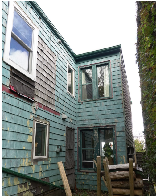
Figure 18: Modifications to back windows (October 23, 2023)
