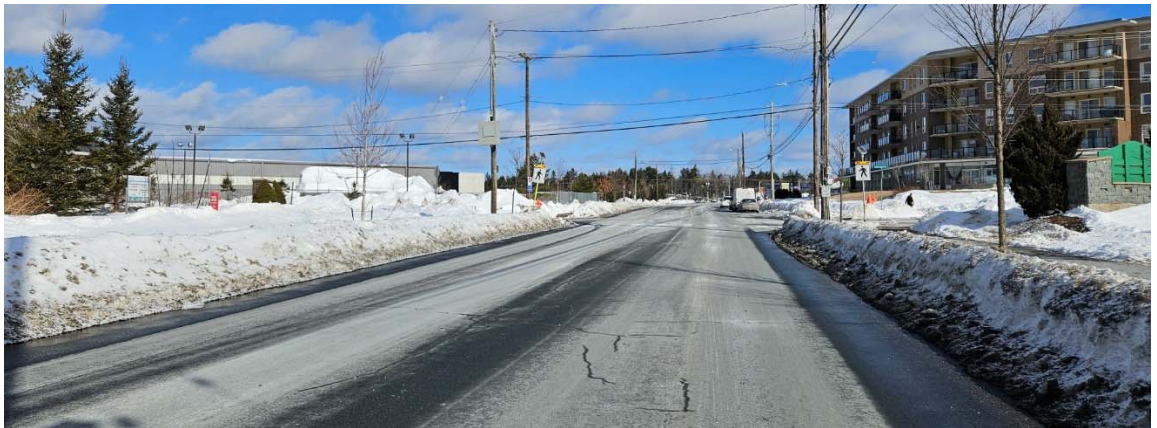
Gary Martin Drive at Innovation Drive/Existing Northwood LTC Driveway looking north
